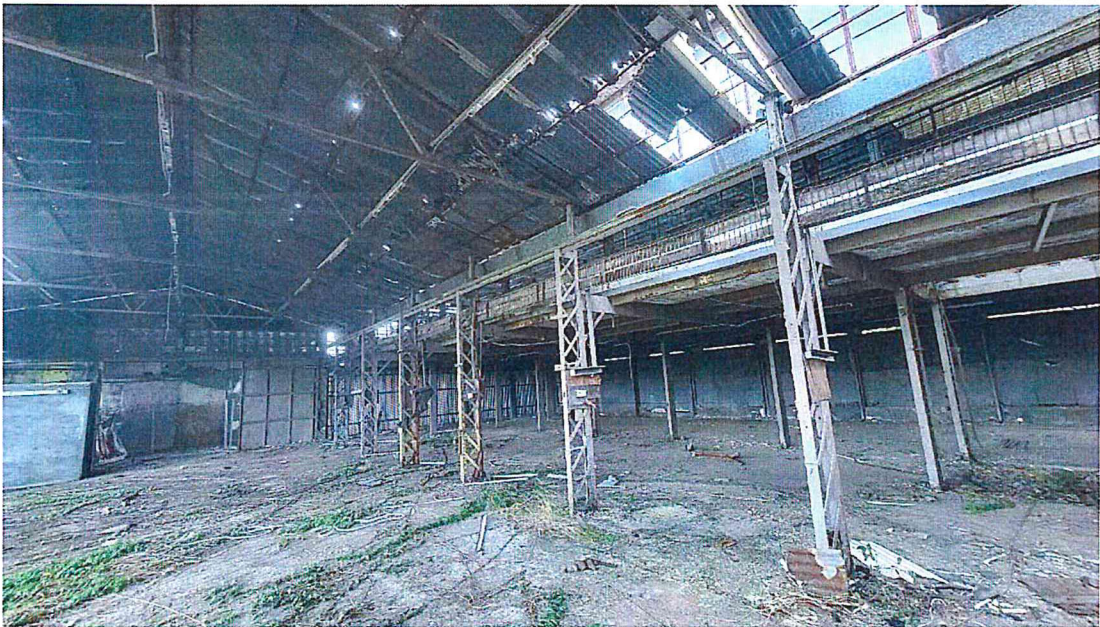
Internal View of an Existing Structure
