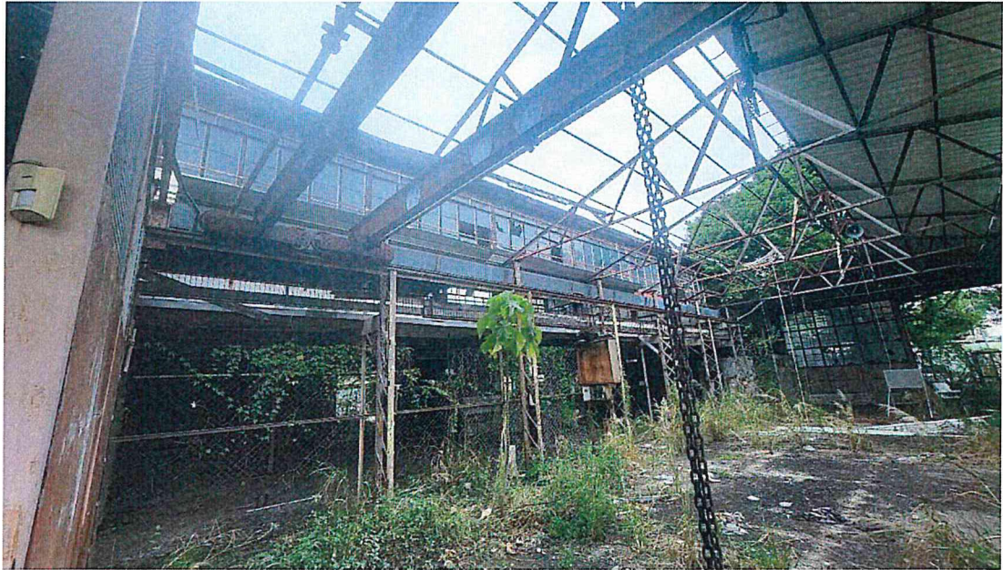
Internal View of an Existing Structure
