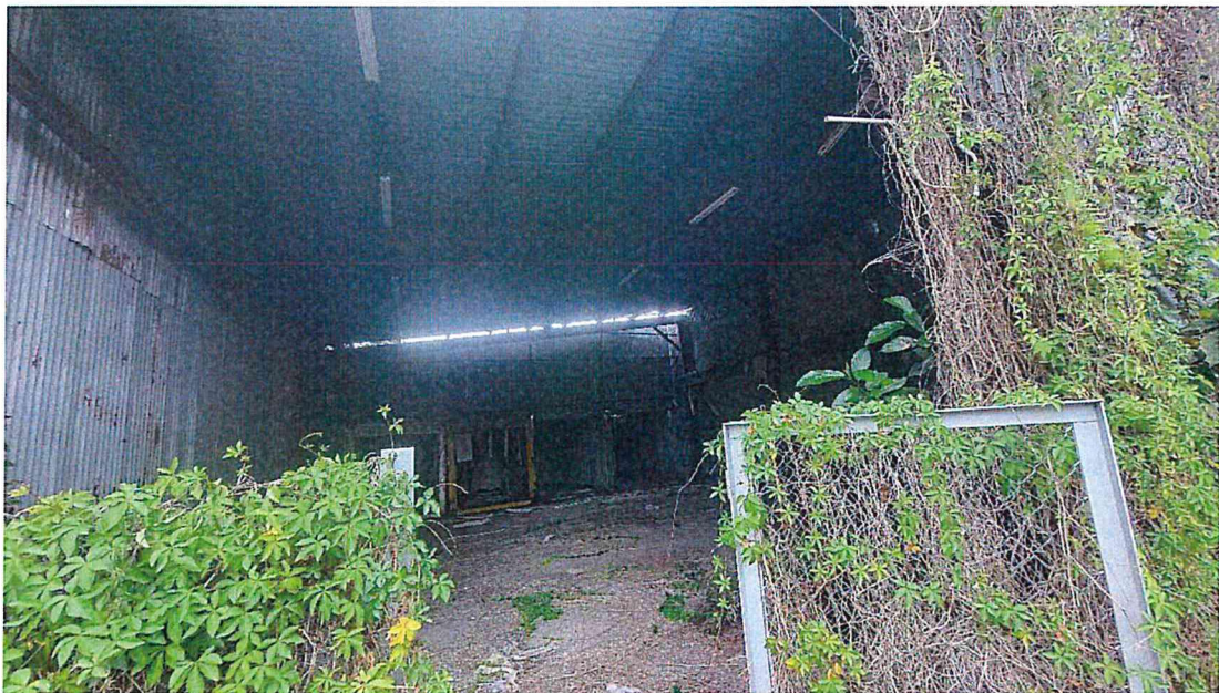
Internal View of an Existing Structure
