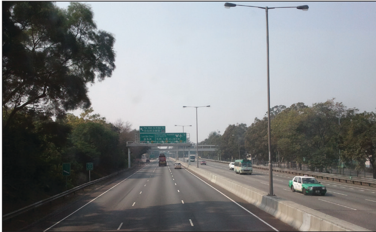
H A prominent linear built element within the landscape is the Fanling Highway.
