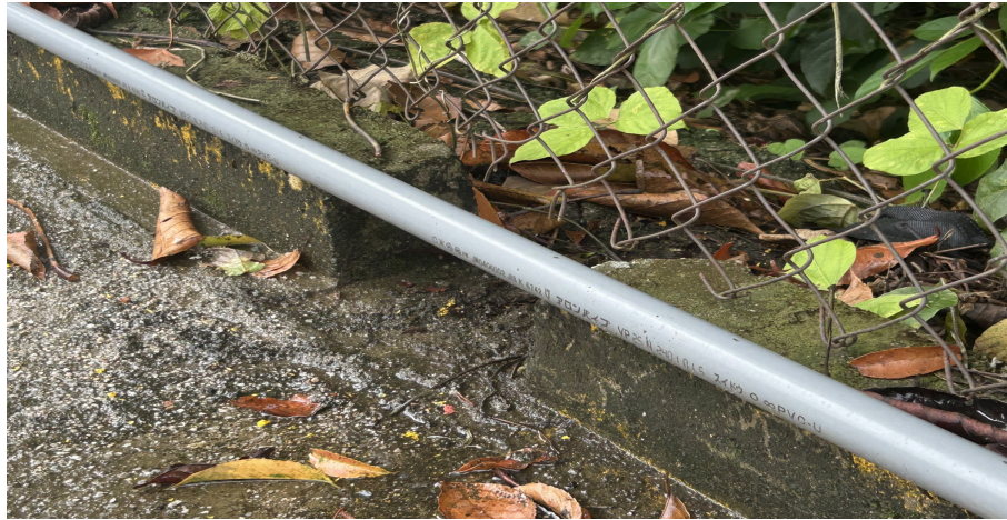
Figure 24: One of the 17 northward drainage outlets at bottom of perimeter fencing
