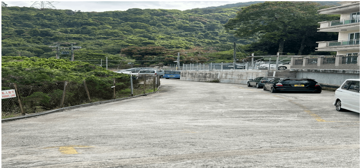
Figure 23: Level and paved concrete of the parking lot
