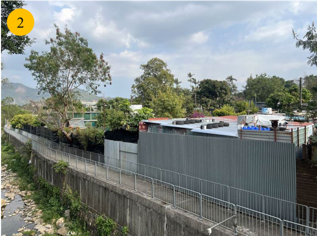
Temporary Structure in Wo Tong Pui next to the Lam Tsuen River under “REC” zone
