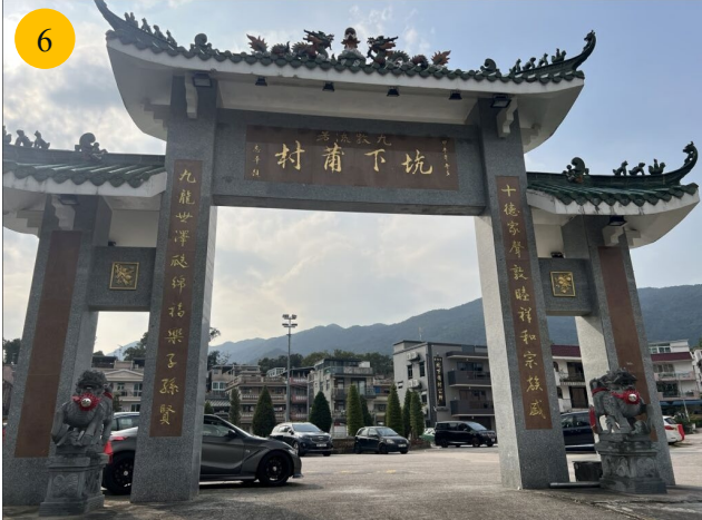
Hang Ha Po Village under “V” zone
