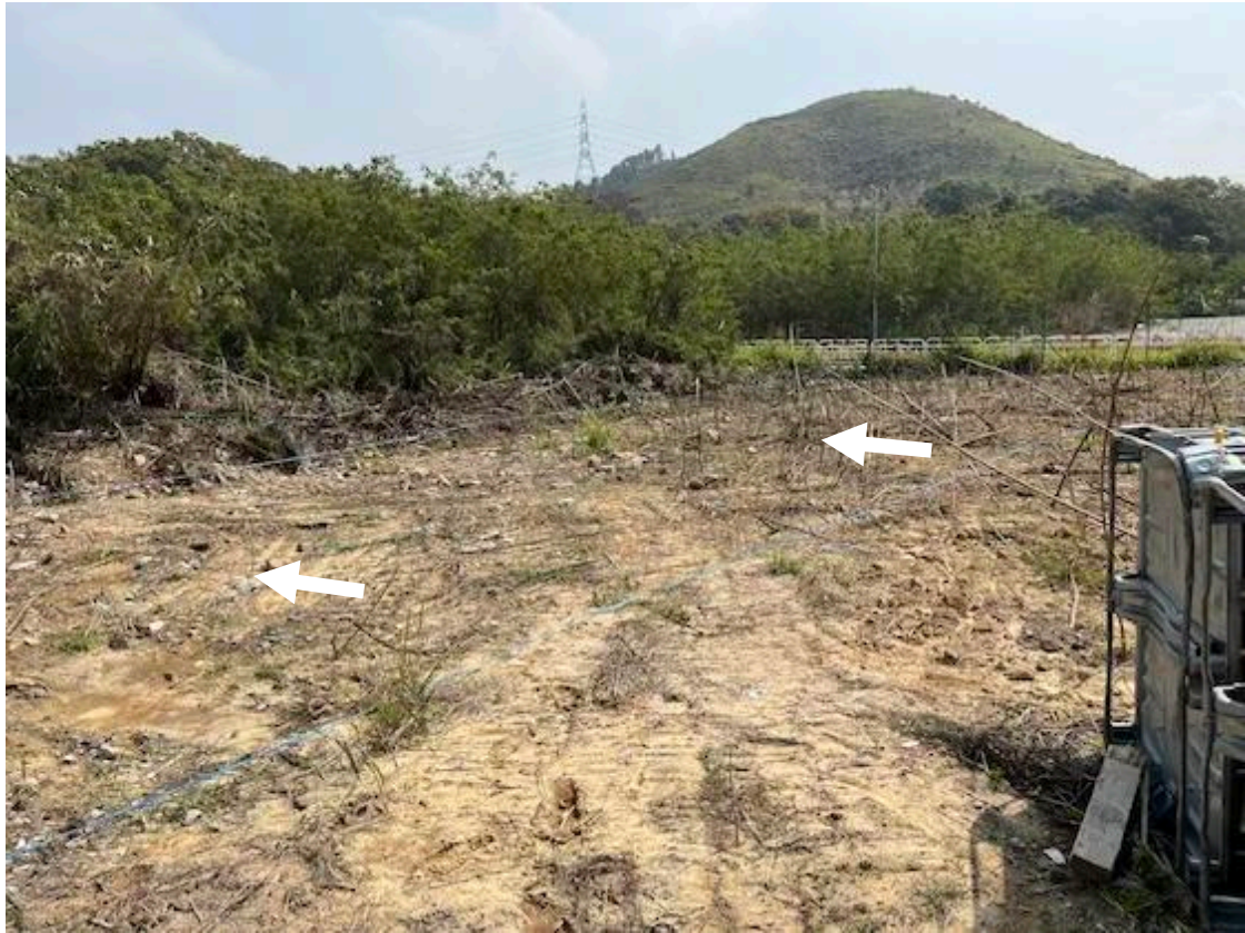
Plate 3 – Existing/original ground sloping away from Site C
