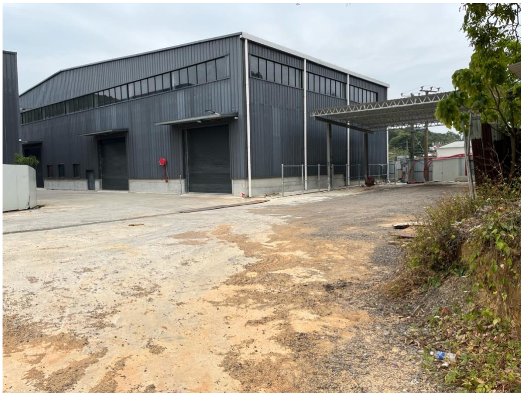
Plate 4 – Existing Site C (December 2023)
