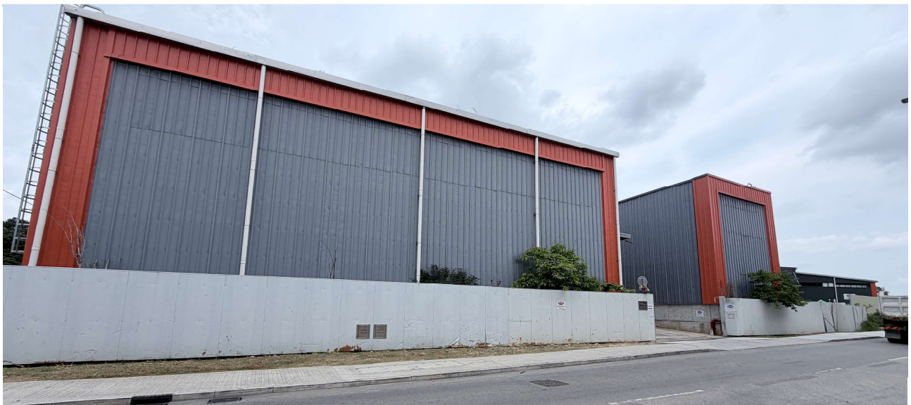
Photo 2: Site C, D, E Entrance
