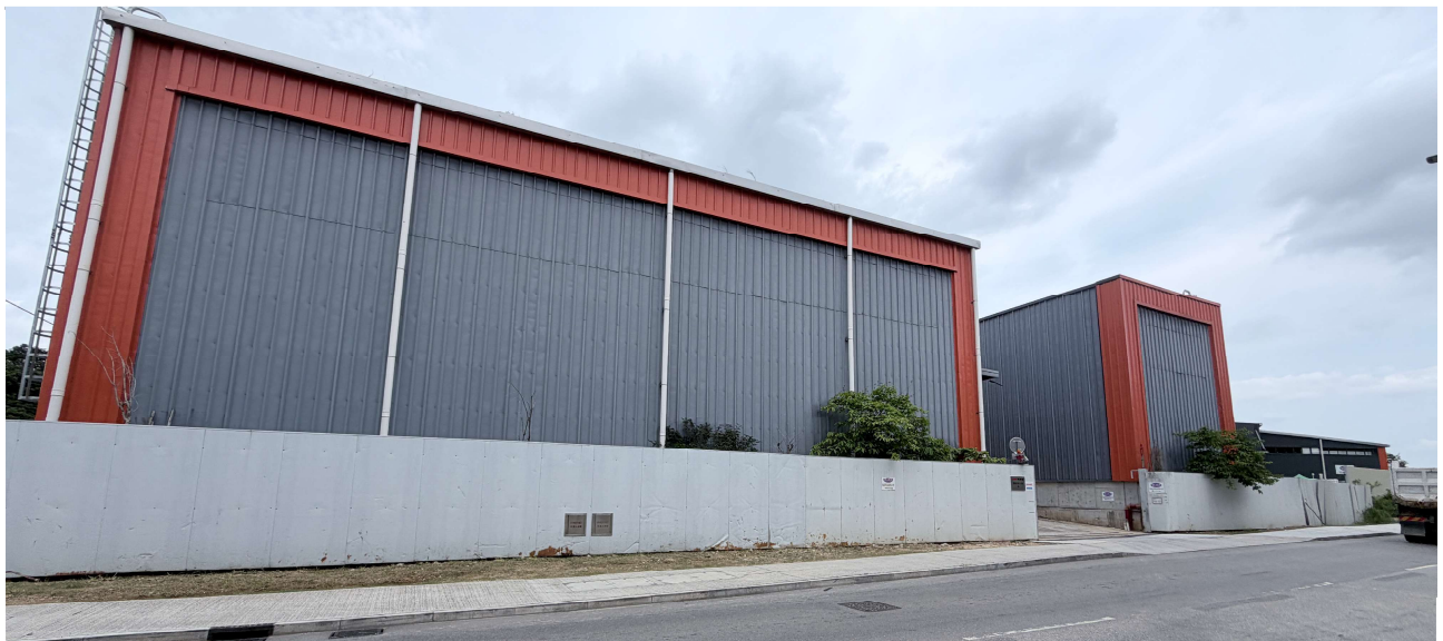
Photo 2: Site C, D, E Entrance
