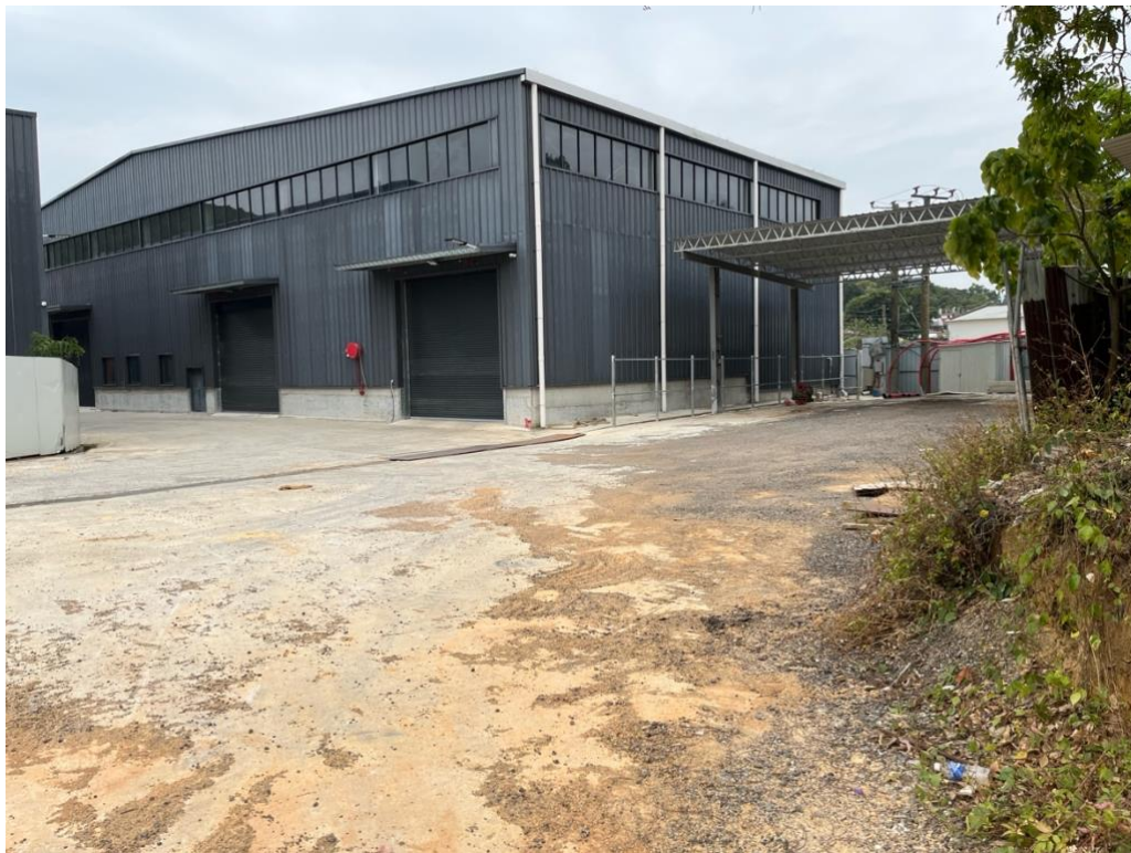
Plate 4 – Existing Site C (December 2023)
