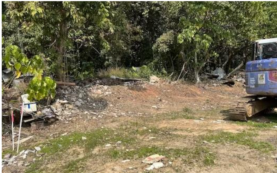
Plate 1 – Small External Catchment (North of Site C)
