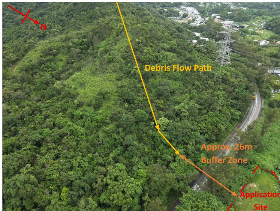
Figure 2 - Aerial view of the Southern side catchment
