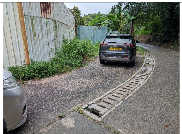
Plate 4 – Existing 300mm u-channel running along the access road outside the northeastern boundary of the Application Site (1 of 2)
