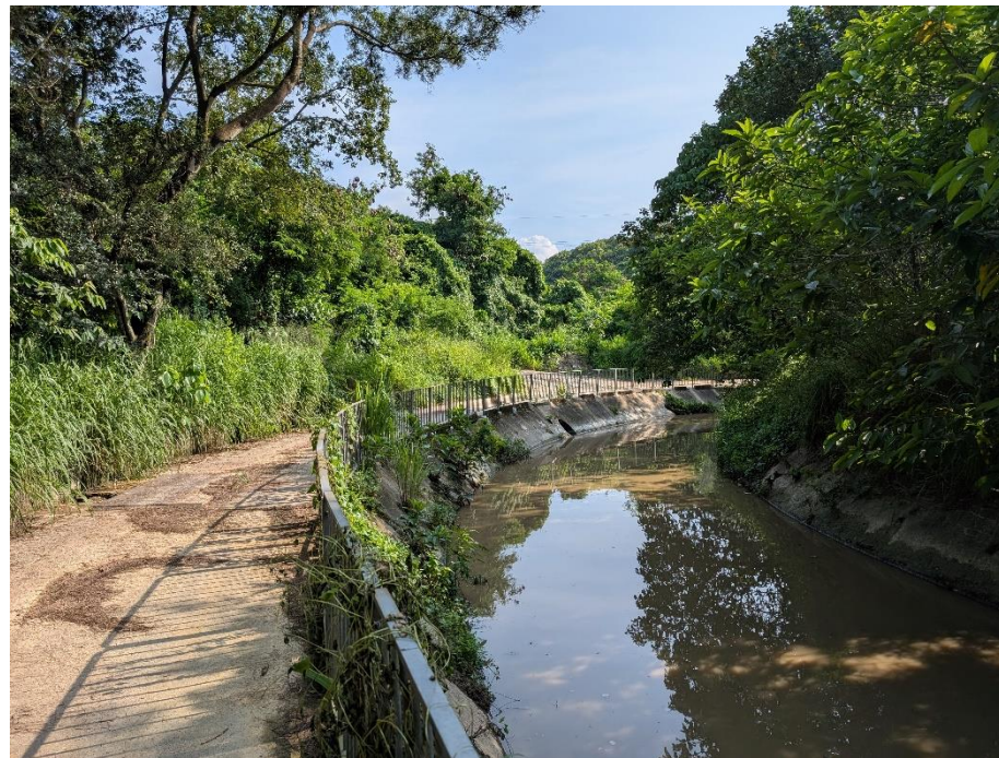
Photo of the existing nullah
