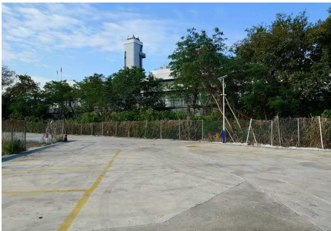
A4 - General view of the site (looking western)
