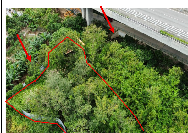
Photo No. 7 – Existing streamcourse running from the east to the west close to the southern boundary of the subject site
