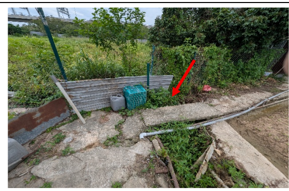
Photo No. 4 – Existing gully receives flow from the drainage ditch of the adjacent farmland and runs across the northern portion of the subject site from the eastern to the western boundary (close-up of the intersection between the drainage ditch of the adjacent farmland and the existing gully)
