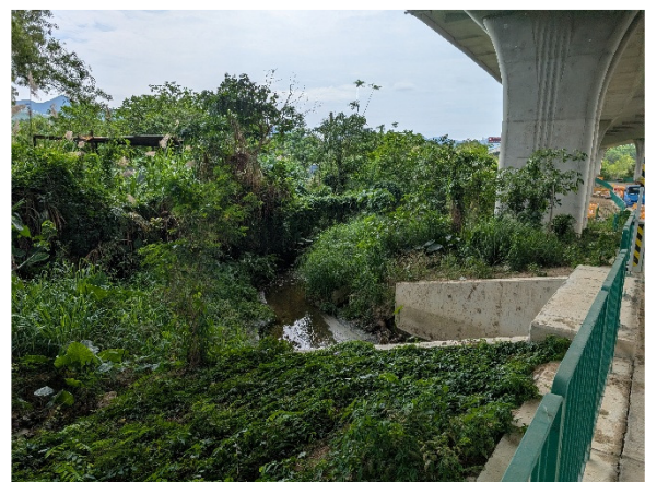
Photo No. 8 – Existing streamcourse and stormwater inlet close to the southern boundary of the subject site under the elevated Heung Yuen Wai Highway from which the flow will pass through twin 900mm diameter drains and go to the west
