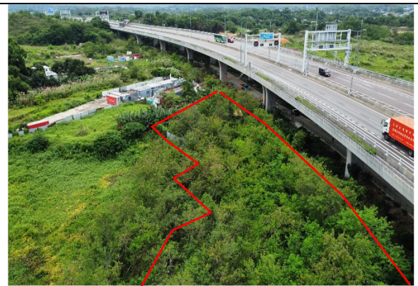
Photo No. 2 – The southern part of the subject site
