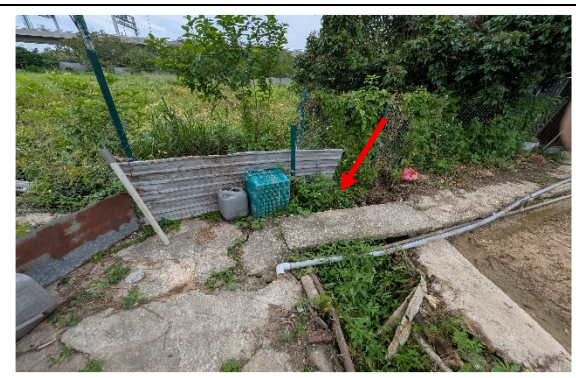
Photo No. 4 – Existing gully receives flow from the drainage ditch of the adjacent farmland and runs across the northern portion of the subject site from the eastern to the western boundary (close-up of the intersection between the drainage ditch of the adjacent farmland and the existing gully)
