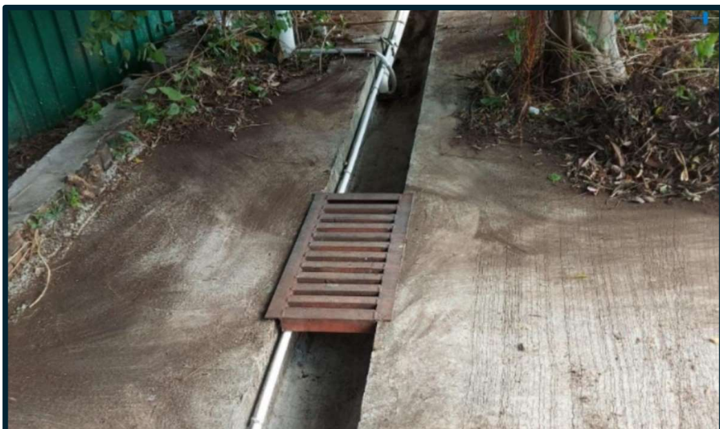
Typical Steel Grating on existing U-channels
