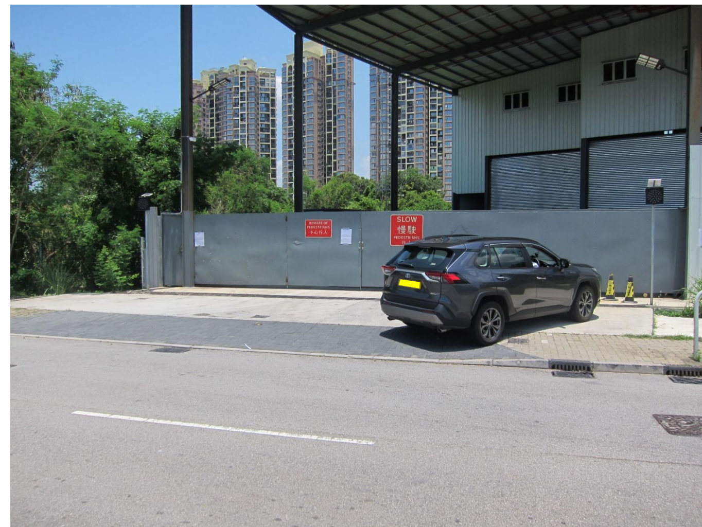
Revolving lights at the entrance
