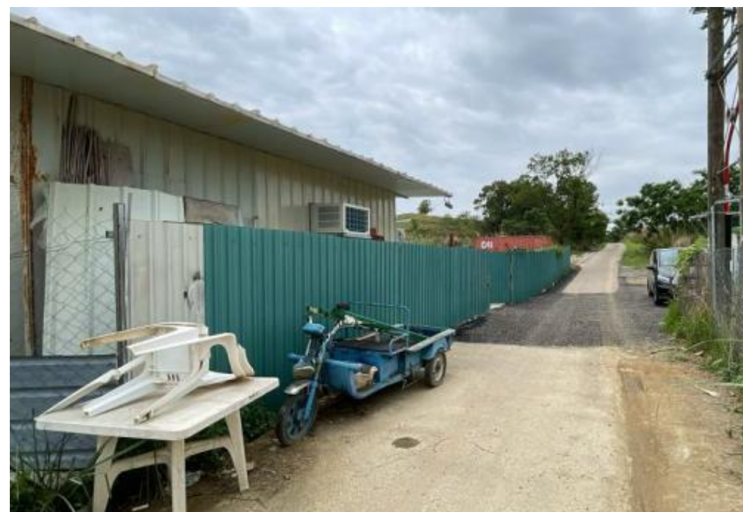
A2 - Temporary Structure Near the South of the Project Boundary (At viewpoint VP4)
