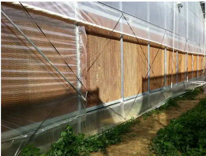
Reference for greenhouse Cooling Pad System 溫室水簾系統參考
