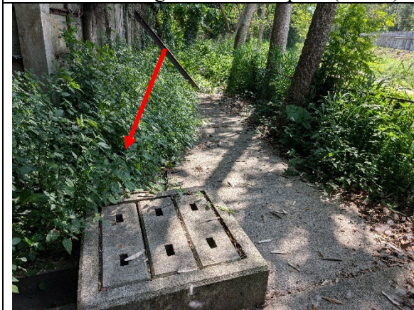
Plate 11 – Existing 300mm U-channel (currently covered up by overgrown with weeds) running between the northern subject site boundary and an existing external footpath (1 of 2)
