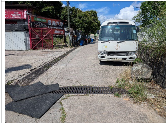
Plate 5 – Existing 450mm U-channel running westward along the existing access in front of the southern subject site boundary (1 of 2)
