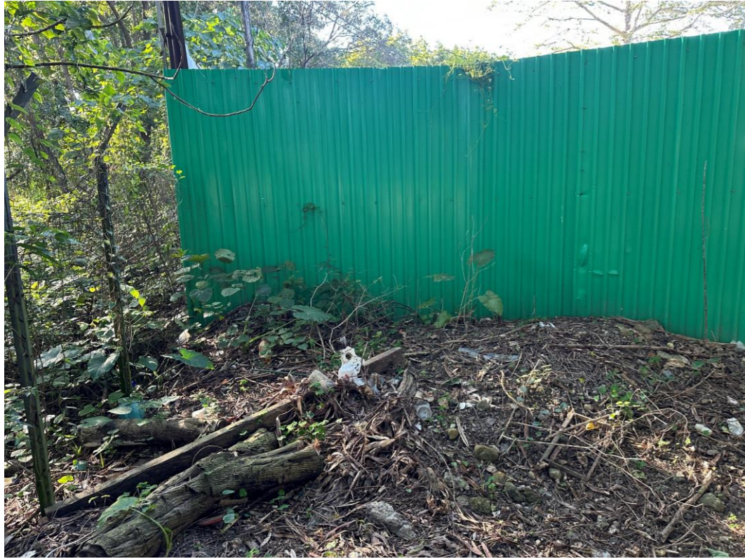
Photo 1: Ramp leading from hoarding of Project Site at southern side
