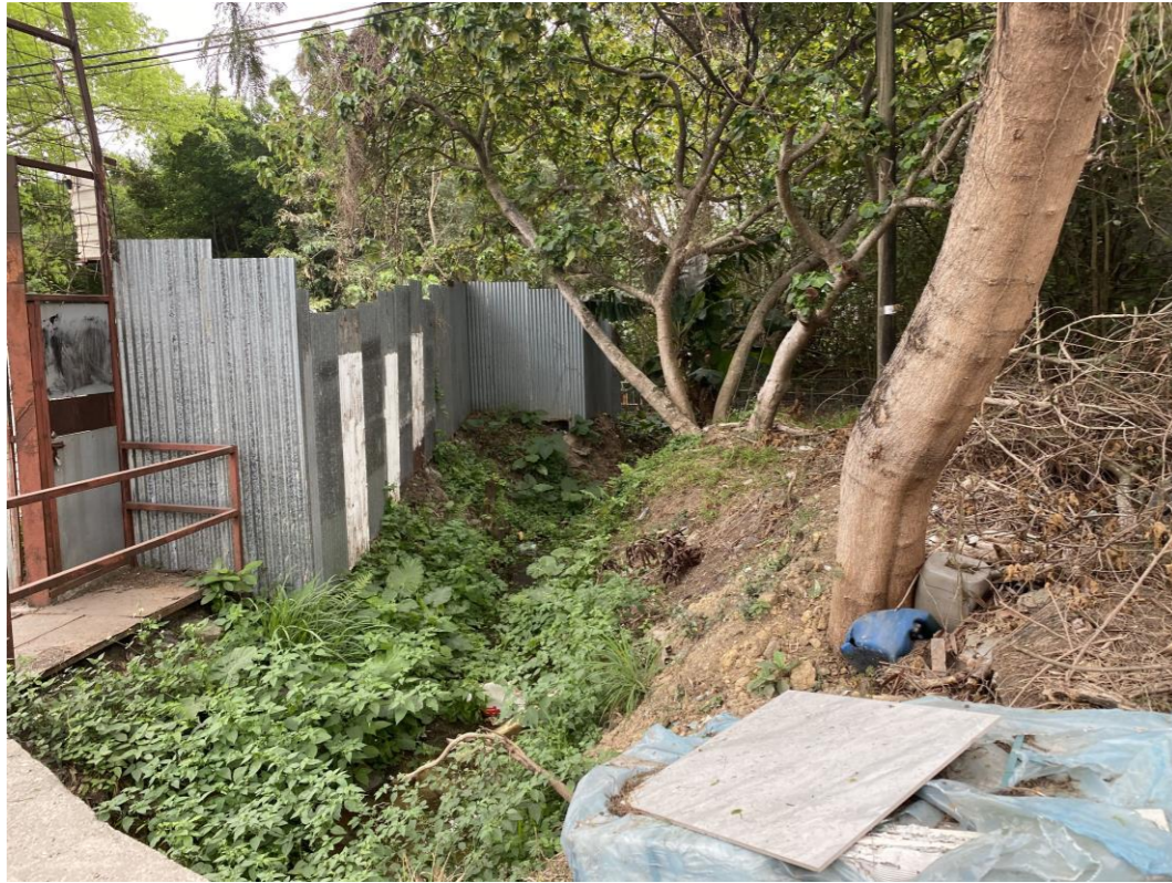
Photo 1: Uncharted U-Channel at the Entrance of the Project Site
