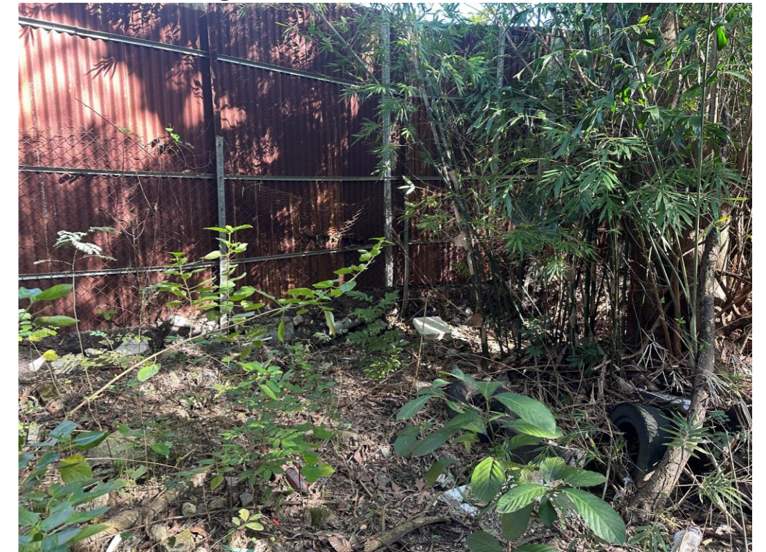
Photo 2: Ramp leading from hoarding of Project Site at western side
