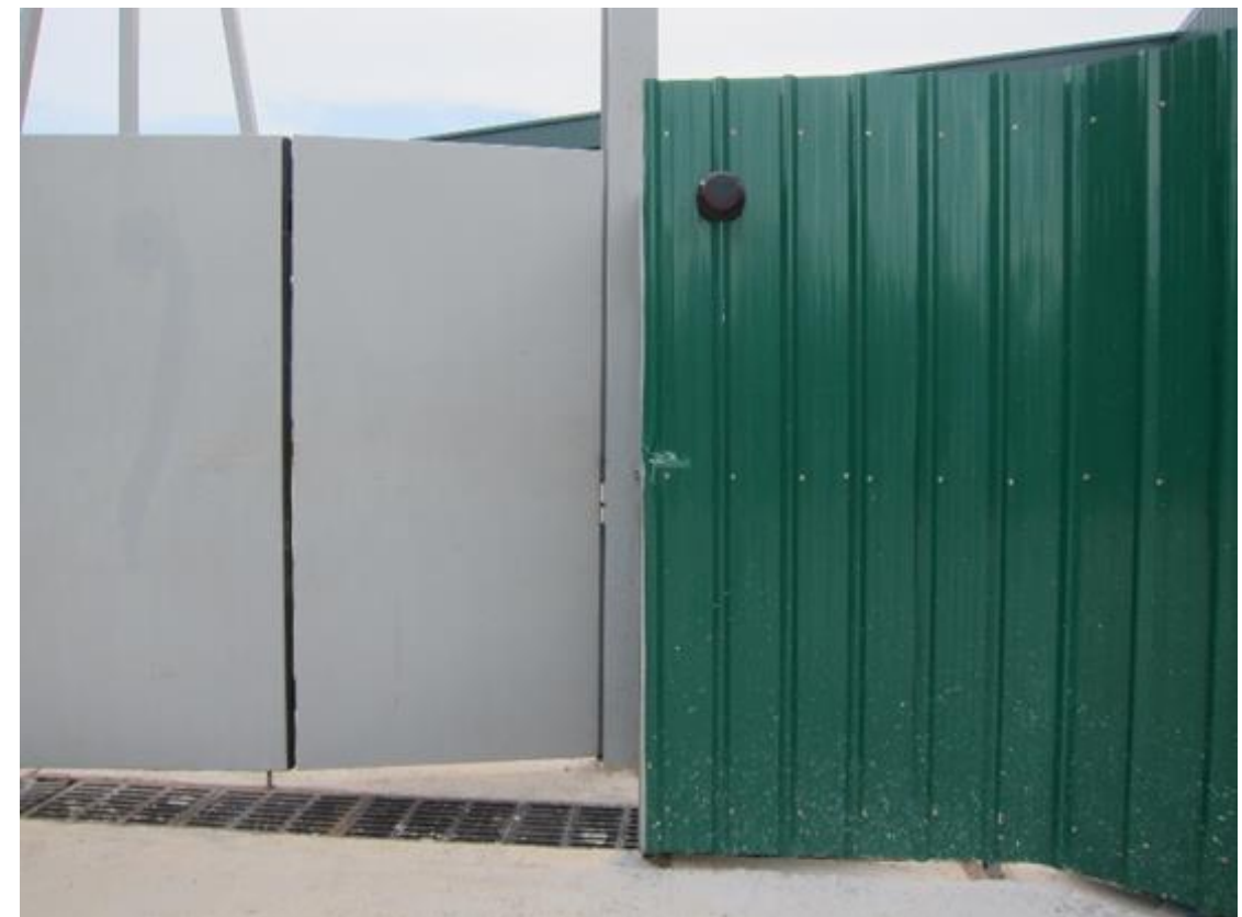
Revolving warning light at right side of the entrance
