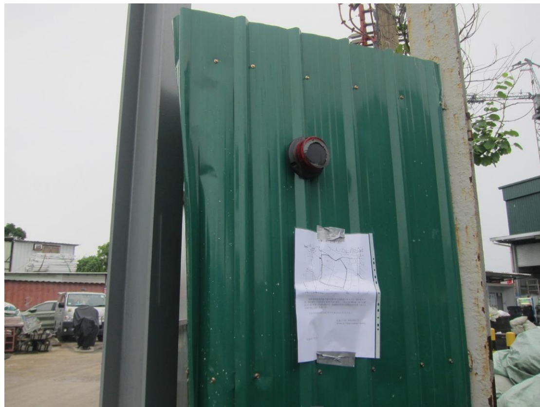
Revolving warning light at left side of the entrance
