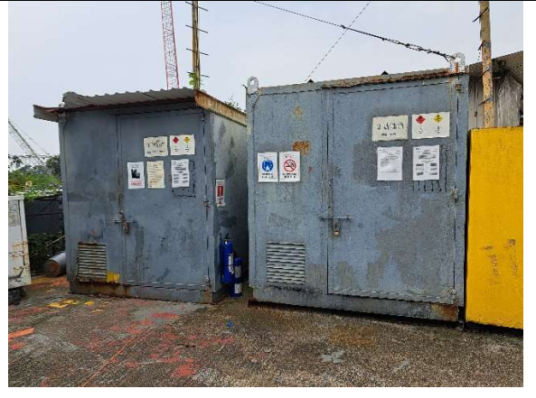
Photo 12: Chemical Storage Area
