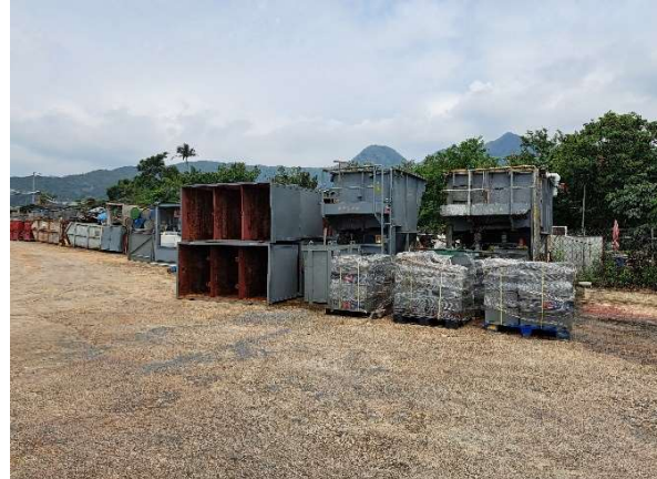
Photo 10: Construction Material Storage
