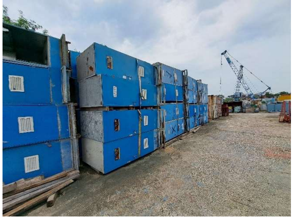
Photo 9: Construction Material Storage
