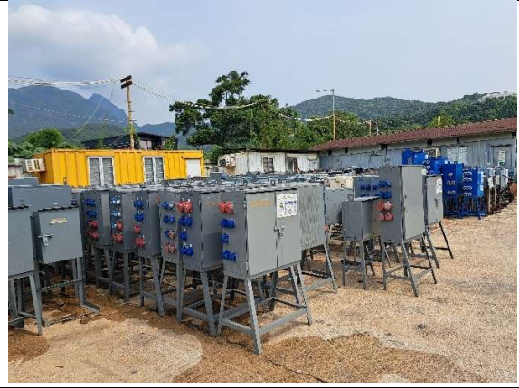
Photo 2: Construction Material Storage
