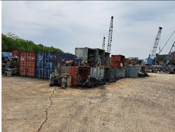
Photo 11: Construction Material Storage
