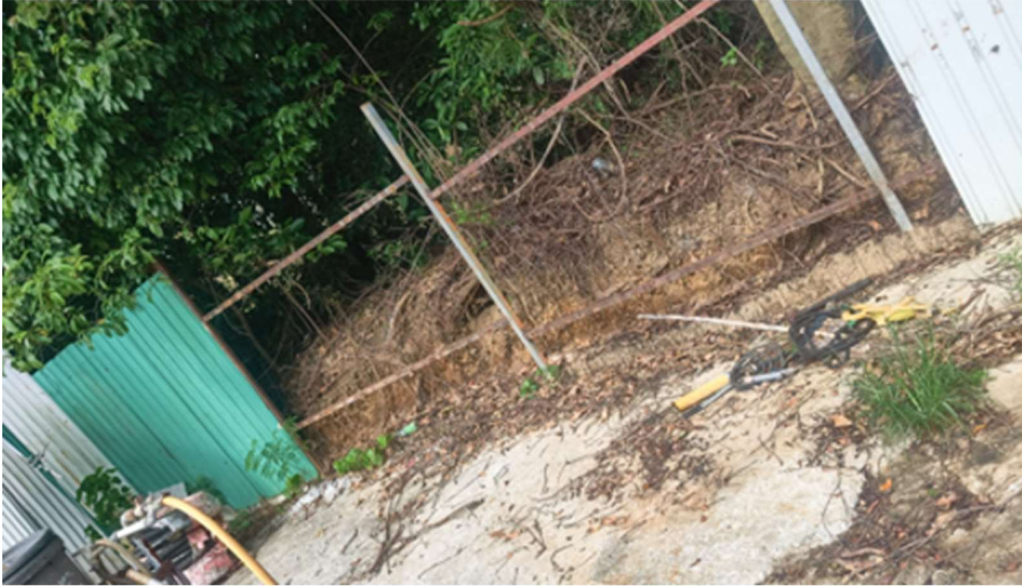
Fences & Hoardings removed
