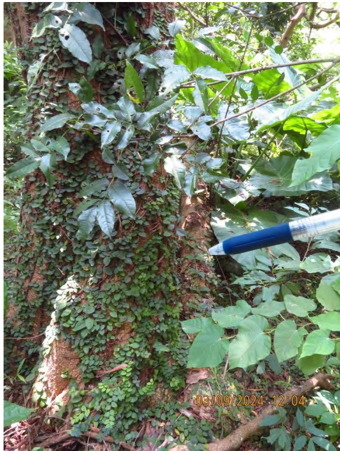
Root flare condition
