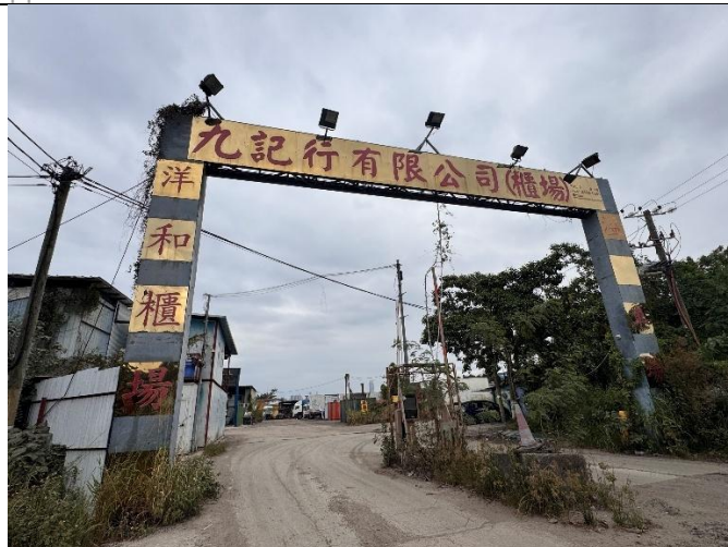
Photo 1: It is the entrance of the open storage. The road is paved with concrete in good condition. No crack and oil stains are observed.
