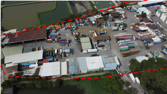
PHOTO W020-2: AERIAL VIEW OF SITE W020
