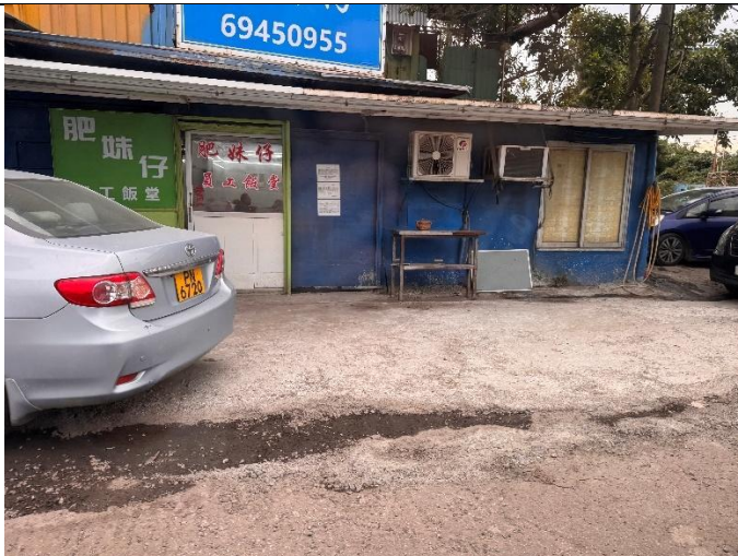
Photo 2: There is a canteen for the staff. The ground is paved with concrete. No crack and oil stains are observed.
