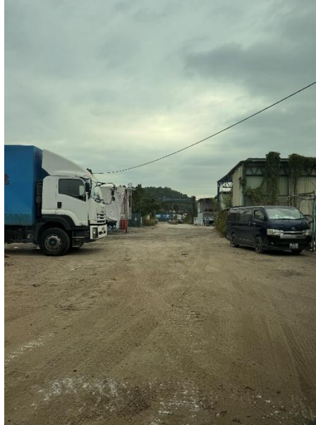
Photo 8: The road is paved with concrete in good condition. No crack and oil stains are observed.
