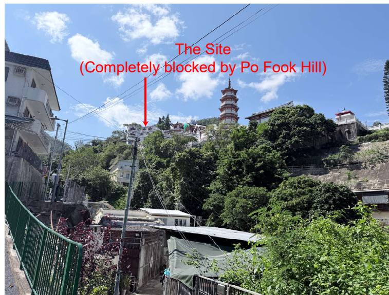
Photo B: View from footpath of Pai Tau Village
