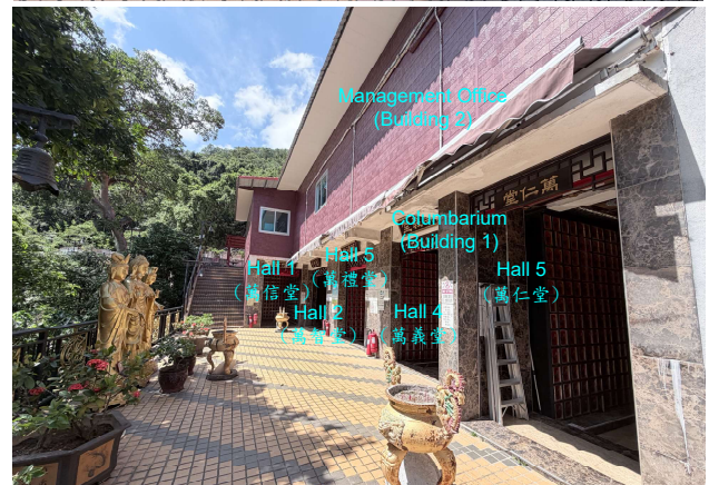
Photo 6: Building 1 and 2 (Ng Sheung Din)
