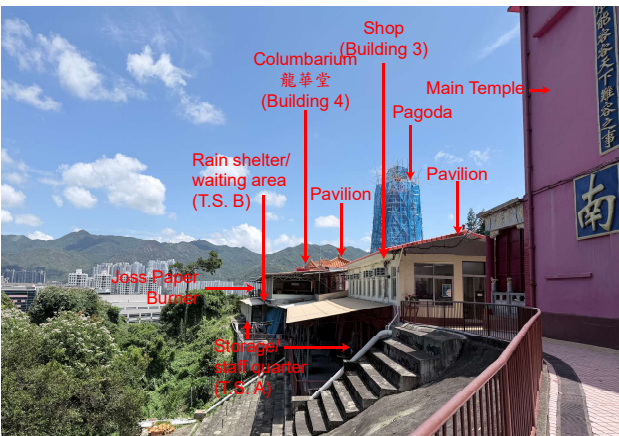
Photo 5: View from northeastern corner of Site A
