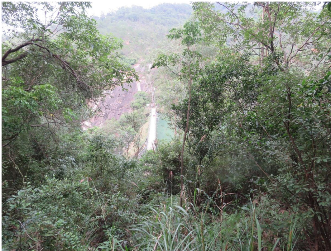
Plate 2 View of reservoir from the Application Site
