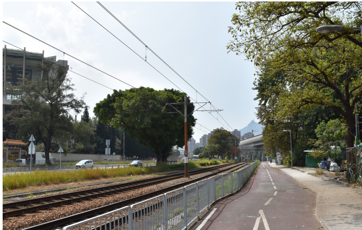
A View south along the LRT Line towards Tuen Mun showing the enclosure formed by a combination of village development and mature tree growth
