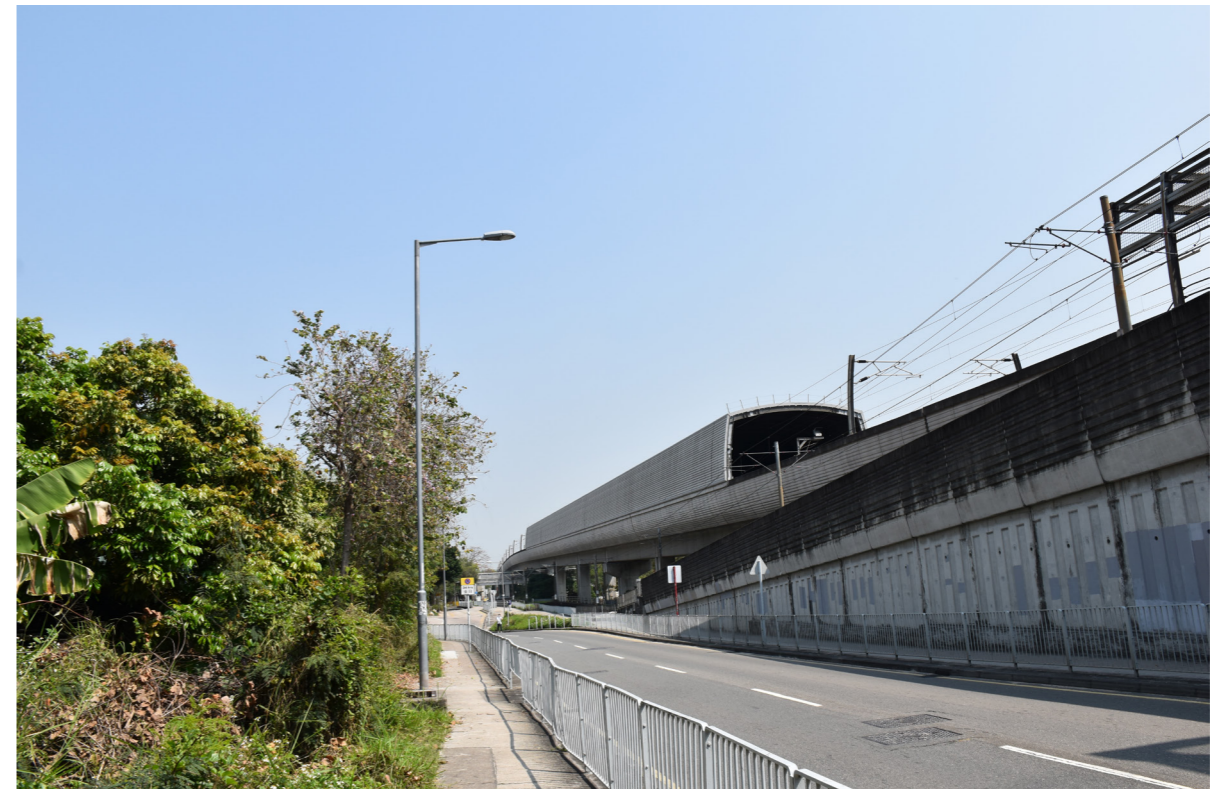
J View looking north demonstrating the visual dominance of the existing infrastructural developments which traverse the village landscape.
