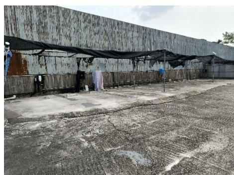
Inflammable mesh will be used as the shelter for the parked vehicle and the charging point
