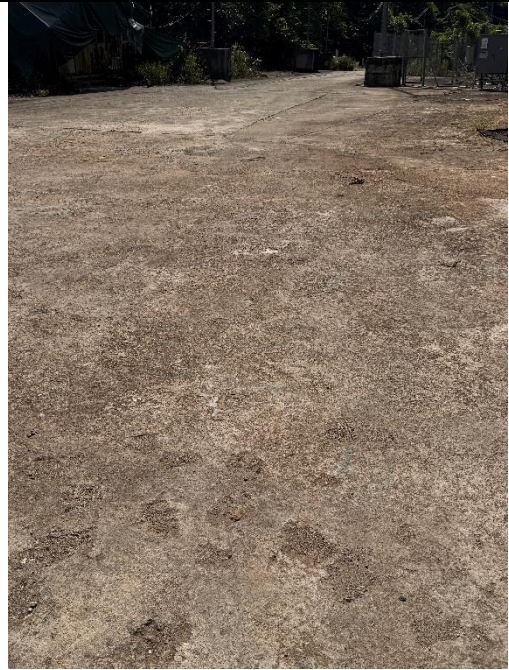
Photo 24: The ground is paved with concrete in good condition
