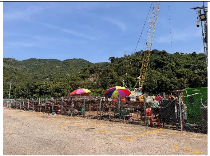
Photo 18: The area is used as temporary storage of construction materials (pile). No chemicals are stored.
