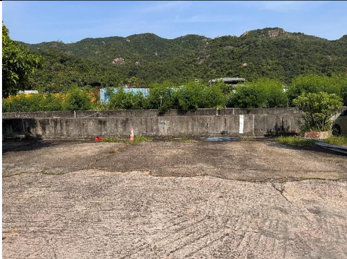
Photo 9: The ground is paved with concrete in good condition. No stains are observed.
