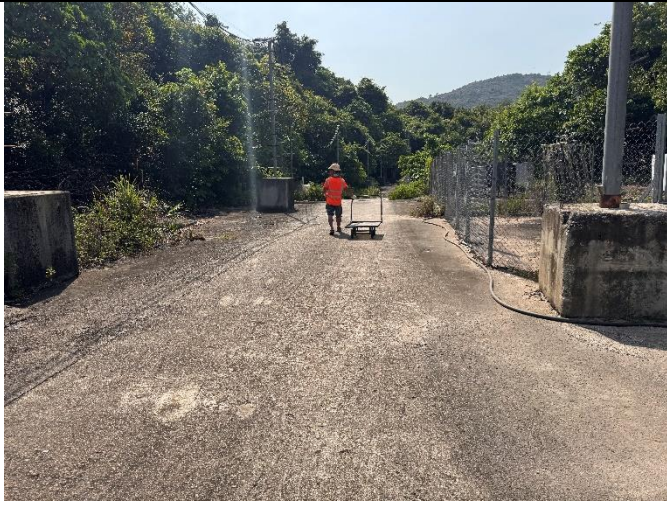
Photo 23: The ground is paved with concrete in good condition
