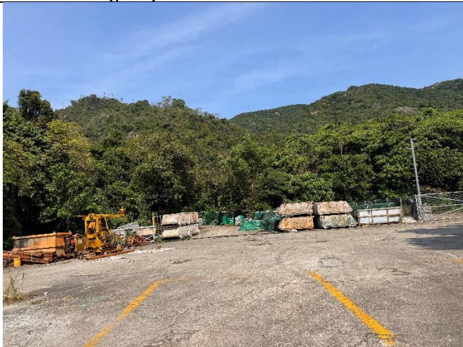
Photo 21: The ground is paved with concrete in good condition. A drill rig is observed but not in operation. Temporary storage is observed. There is no direct contact between the stuff and the ground
