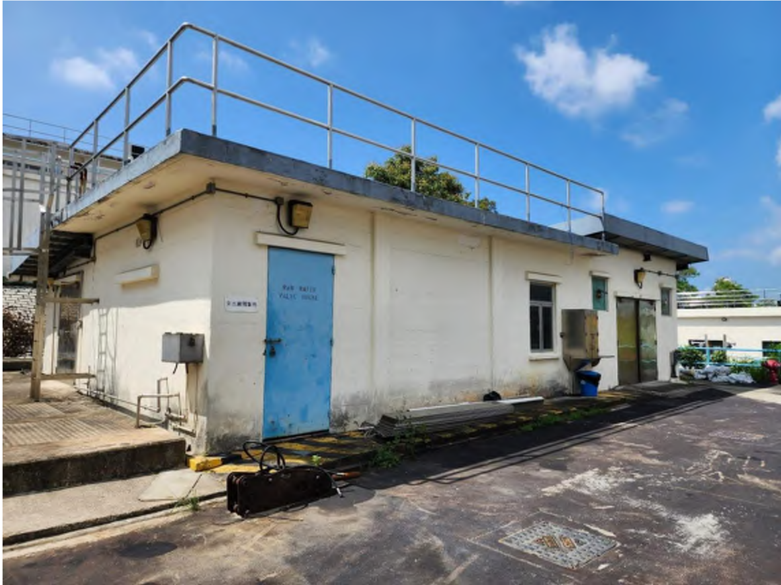
Site Photo 9 - Existing Inlet Valve House and E&M Workshop
