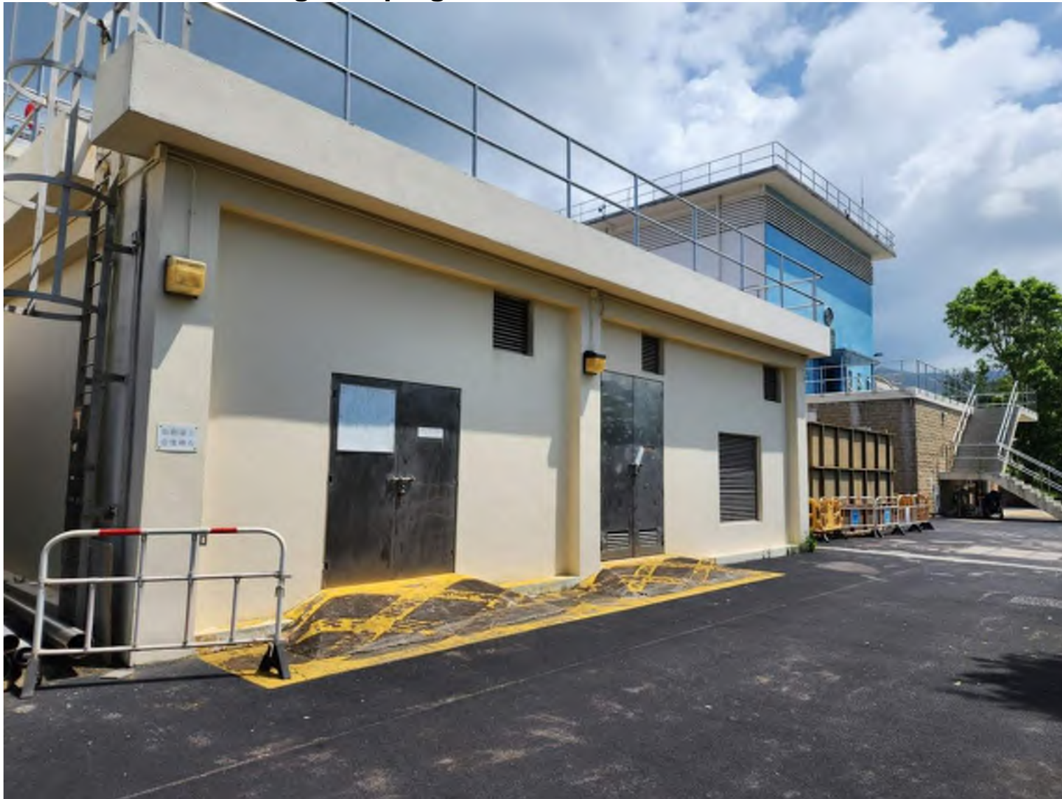
FIGURE 7 Site Photo 2 - Existing Pumping House
