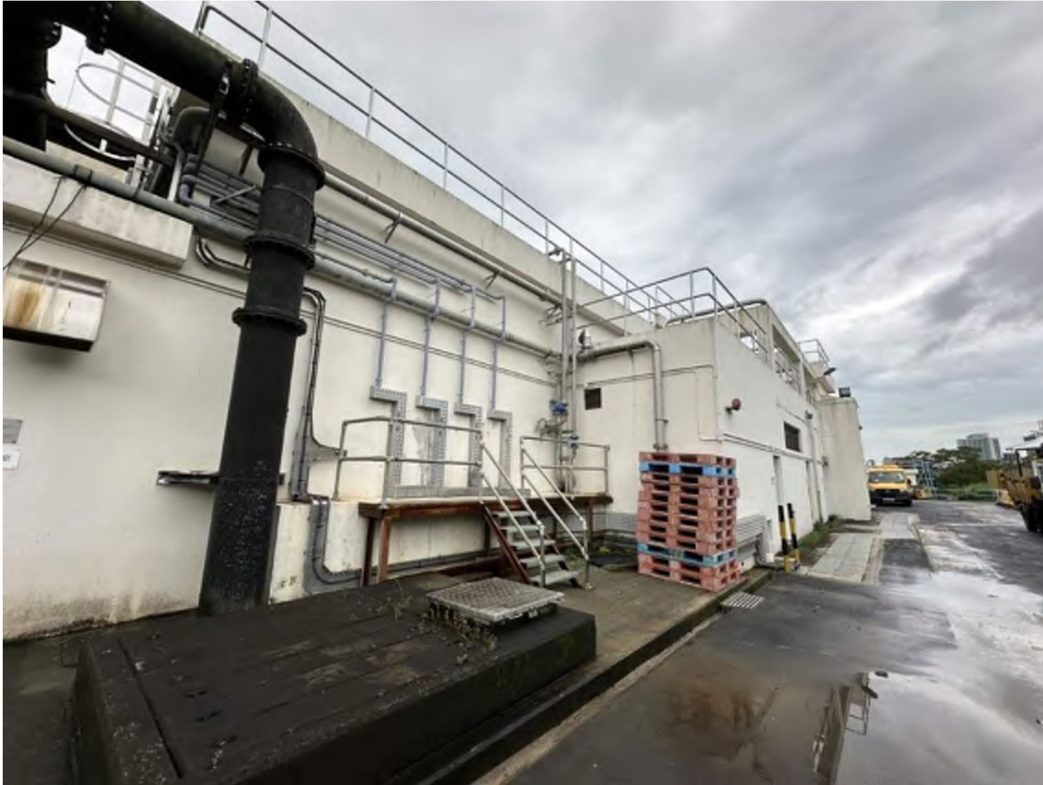
Site Photo 8 - Existing Chlorination House (Not in Used)
