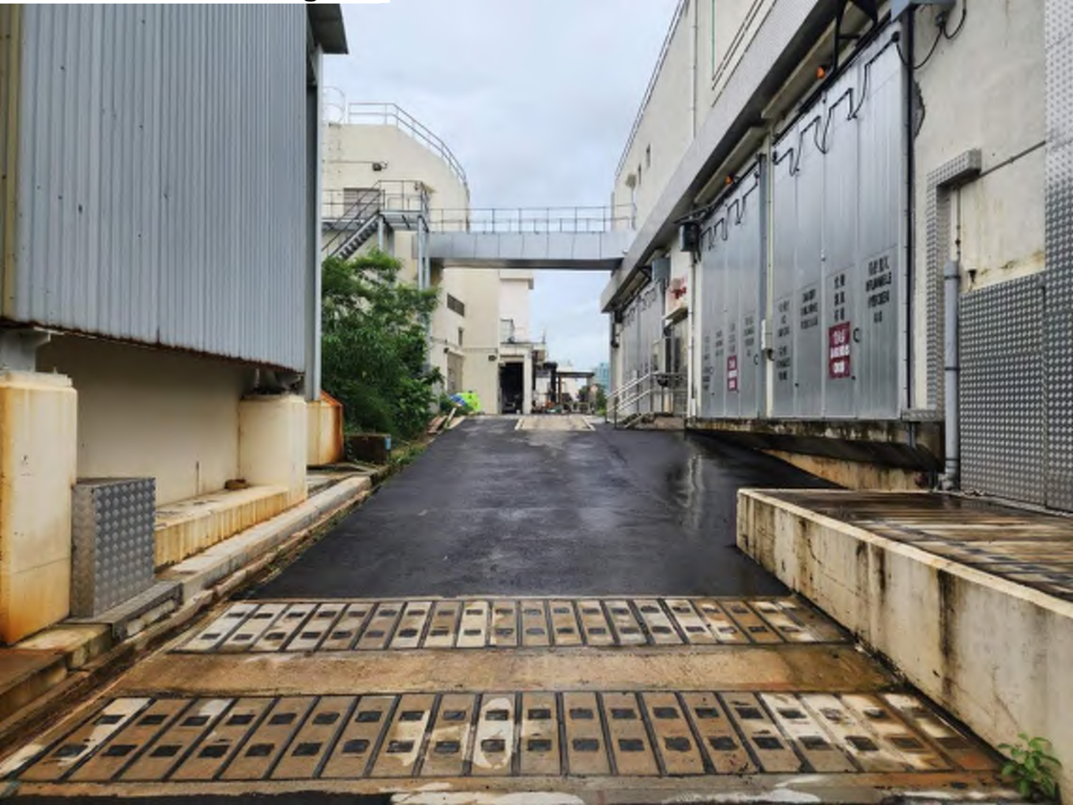
Site Photo 4 - Existing Access Road
