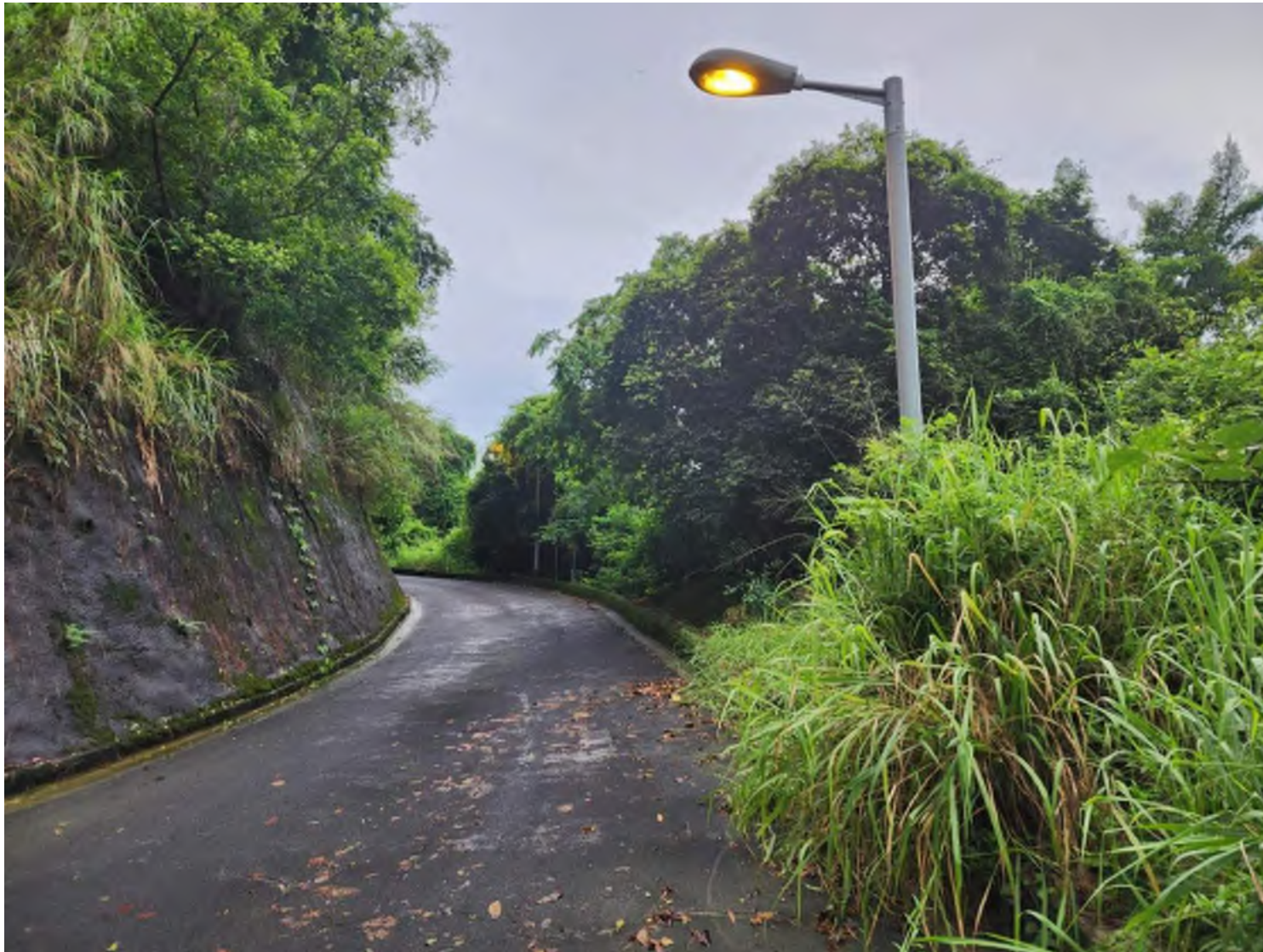
Site Photo 16 - Access Road to TWWTW
