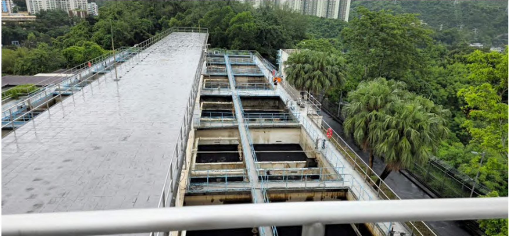
Site Photo 13 - Existing East Wing
