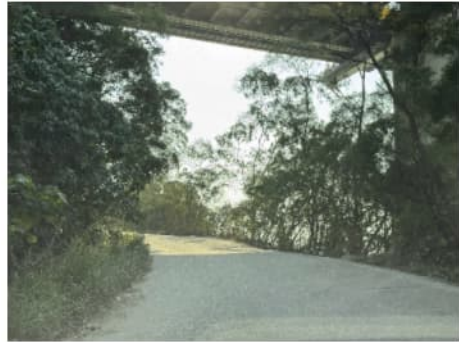
PHOTO 3389: ACCESS ROAD (DATE TAKEN: 8 APRIL 2025)
