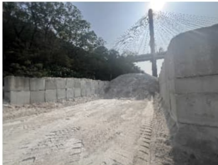
PHOTO 5962: STOCKPILING AREA (DATE TAKEN: 8 APRIL 2025)
