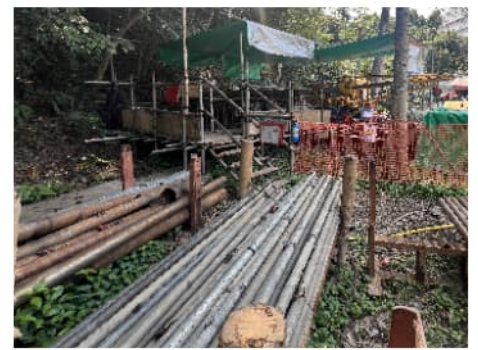
PHOTO 5655: MATERIAL STORAGE AREA FOR DRILL RODS AND ELEVATED WORKING PLATFORM (DATE TAKEN: 8 APRIL 2025)
