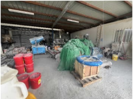
PHOTO 5981: MATERIAL STORE FOR MIST MACHINE AND CHEMICAL STORAGE AREA (DATE TAKEN: 8 APRIL 2025)
