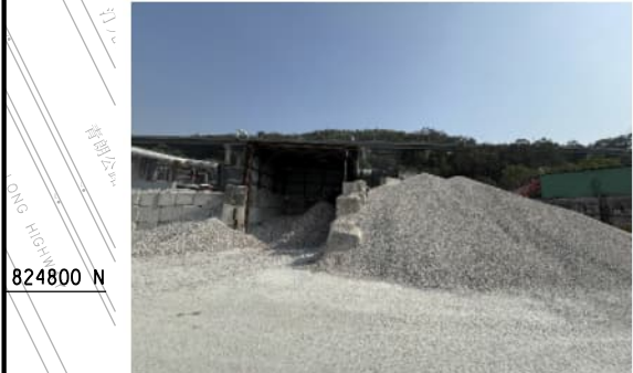
PHOTO 3258: STOCKPILING AREA (DATE TAKEN: 8 APRIL 2025)
