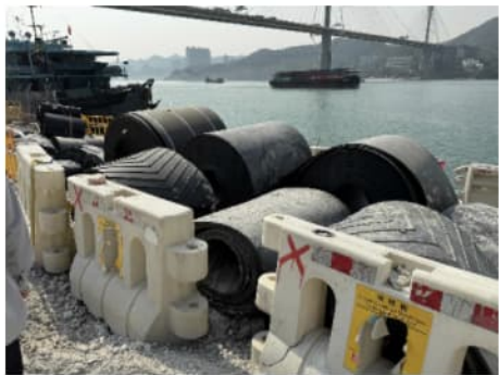
PHOTO 3252: RUBBER CONVEYOR BELTS IN MATERIAL STORAGE AREA (DATE TAKEN: 8 APRIL 2025)
