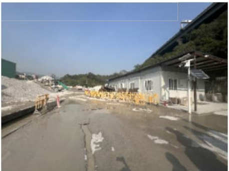
PHOTO 6034: RECORDER HOUSE (DATE TAKEN: 8 APRIL 2025)
