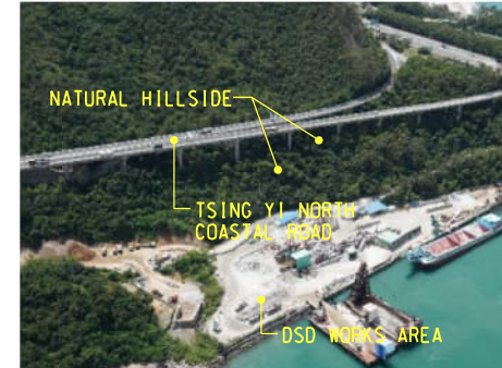
PHOTO 0318: DSD WORKS AREA OF CONTRACT NO. DC/2020/05 RELOCATION OF SHA TIN SEWAGE TREATMENT WORKS TO CAVERNS - MAIN CAVERNS CONSTRUCTION AND NATURAL HILLSIDE (DATE TAKEN: 18 SEPTEMBER 2023)
