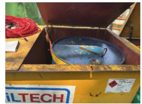
PHOTO 5664: DIESEL OIL IN CHEMICAL STORAGE CABINET (DATE TAKEN: 8 APRIL 2025)
