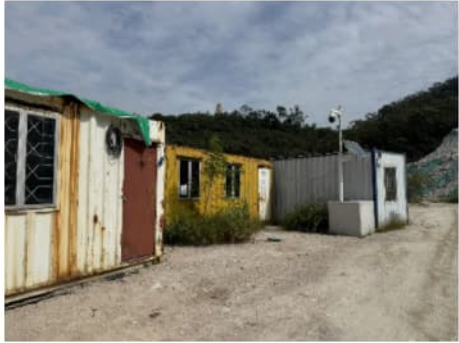
PHOTO 0349: REST ROOM (DATE TAKEN: 20 OCTOBER 2025)
