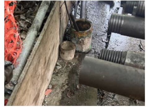
PHOTO 5649: LUBRICATING OIL ON WOODEN PLANK OF AN ELEVATED WORKING PLATFORM WITH WOODEN SIDEBOARDS (DATE TAKEN: 8 APRIL 2025)
