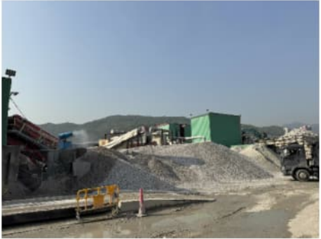
PHOTO 3338: WEIGHBRIDGE, STOCKPILING AREA AND CRUSHING AND SCREENING FACILITIES (DATE TAKEN: 8 APRIL 2025)
