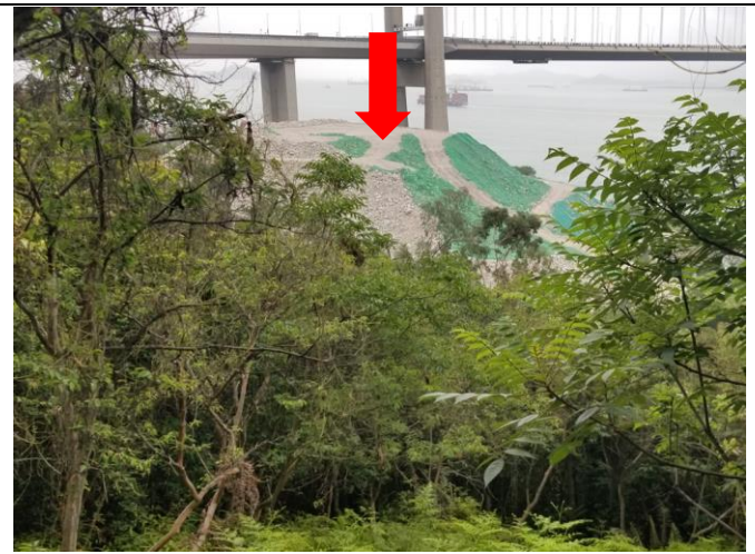
Wok Tai Wan Works Area (Developed Area)
