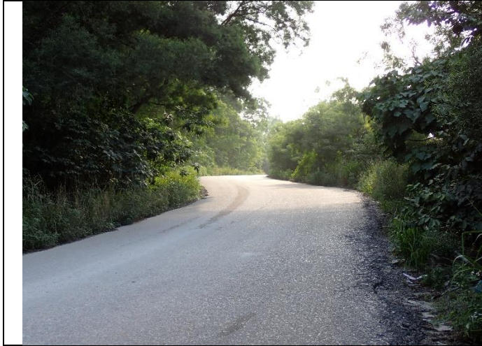
Access Road west of Ngau Kok Wan Portal
