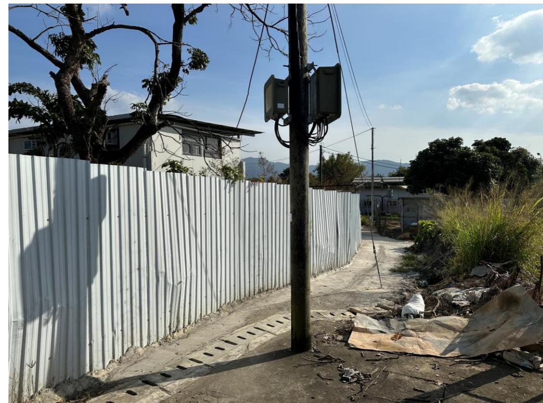
Photo 3: Hoarding with Concrete Footing
