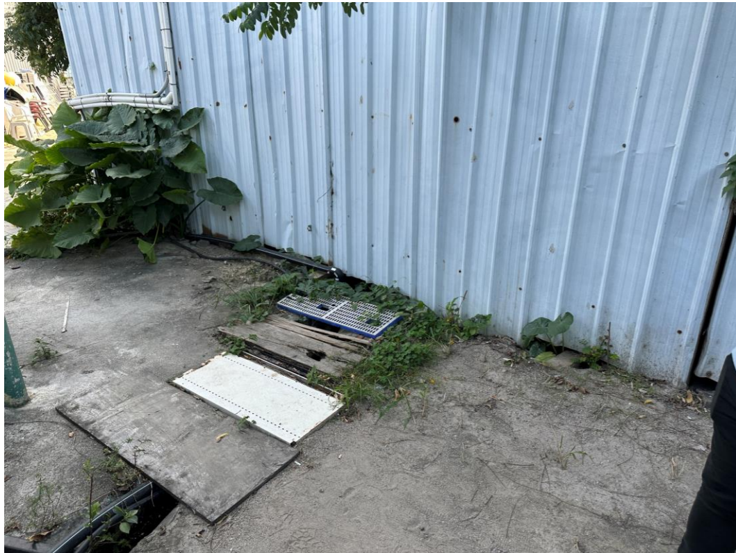
Photo 1: Hoarding without concrete footing
