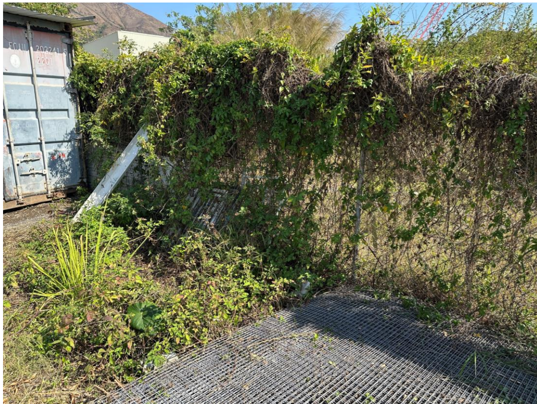
Photo 2: Hoarding without Concrete Footing
