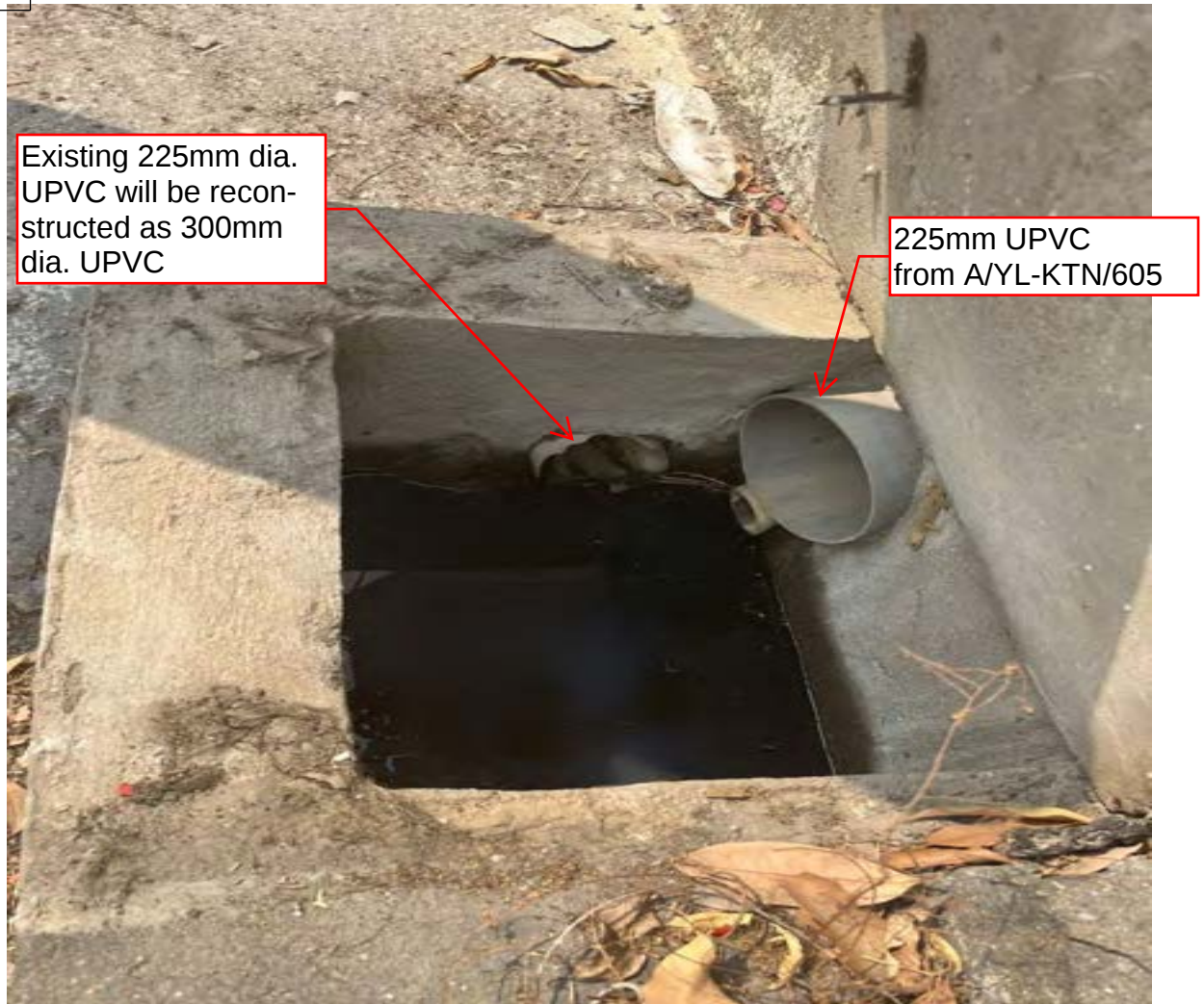
Existing Condition of CP4 and existing 225mm dia. pipe
