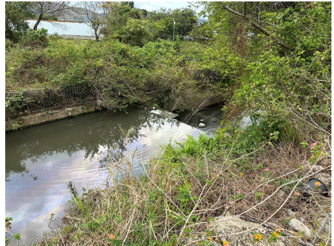
Photo 3: Stepped Channel at South of the Project Site
