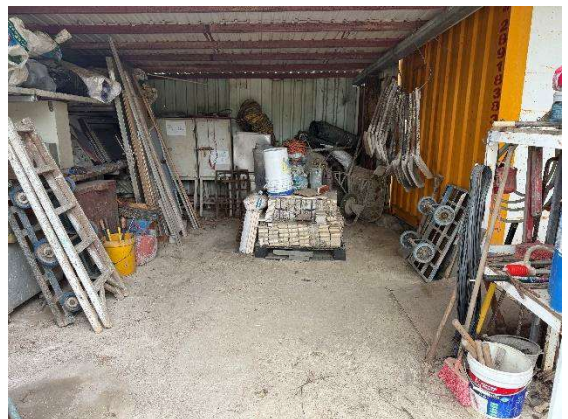
Photo 12: Temporary storage of construction equipment / tools within the temporary structure
