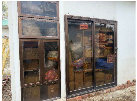
Photo 4: South: Temporary structure at western side of the existing residential house for domestic storage
