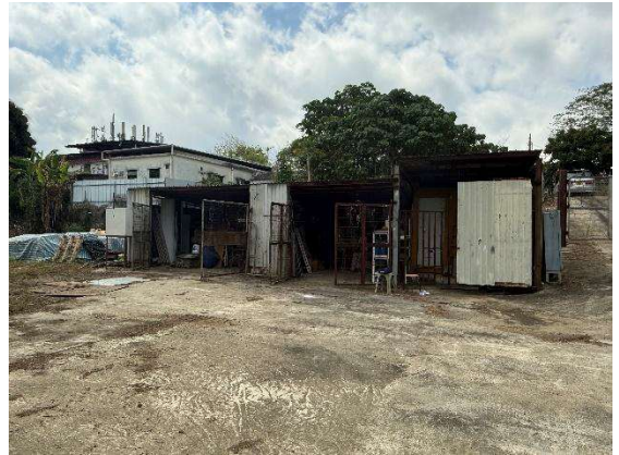
Photo 10: South East: Temporary structure for storage of construction equipment and material
