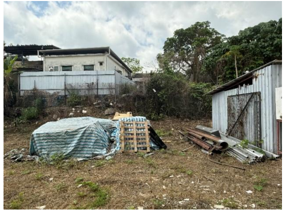
Photo 14: Temporary storage of steel bars and tiles
