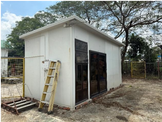
Photo 3: South: Temporary structure at western side of the existing residential house for domestic storage
