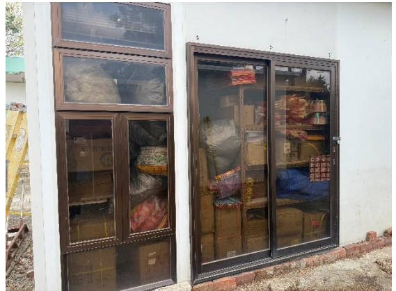
Photo 4: South: Temporary structure at western side of the existing residential house for domestic storage
