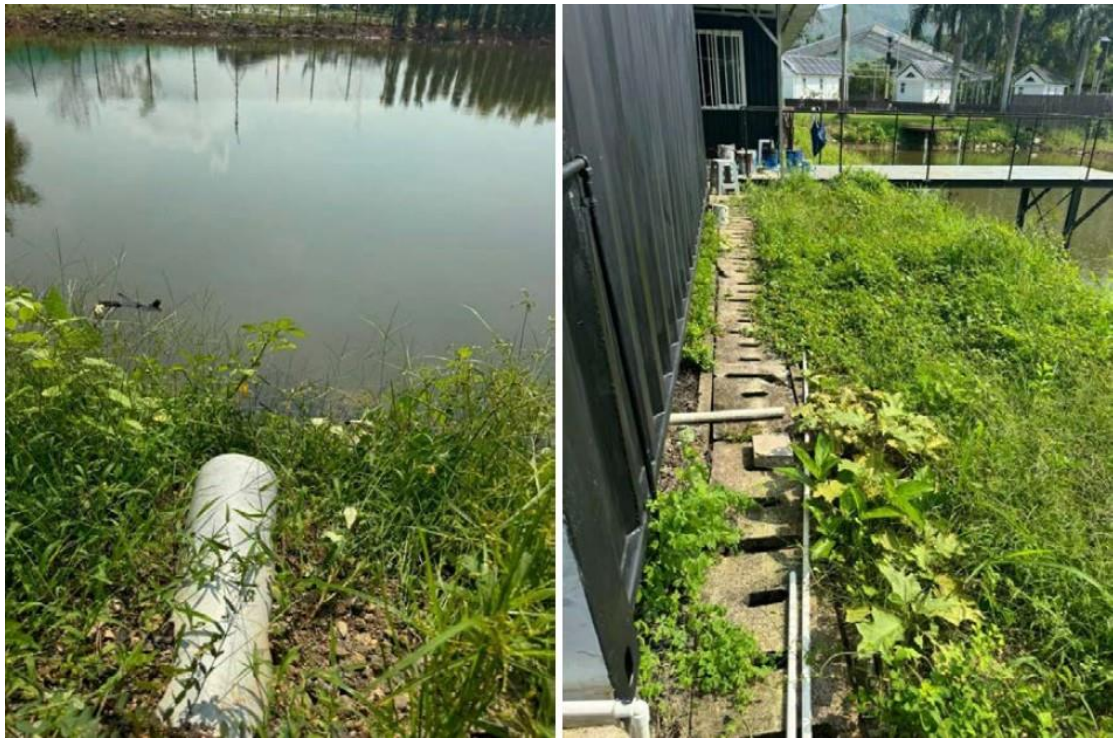
P6 & P7 Existing Pond at Lot 21 in DD109 for collecting Stormwater
