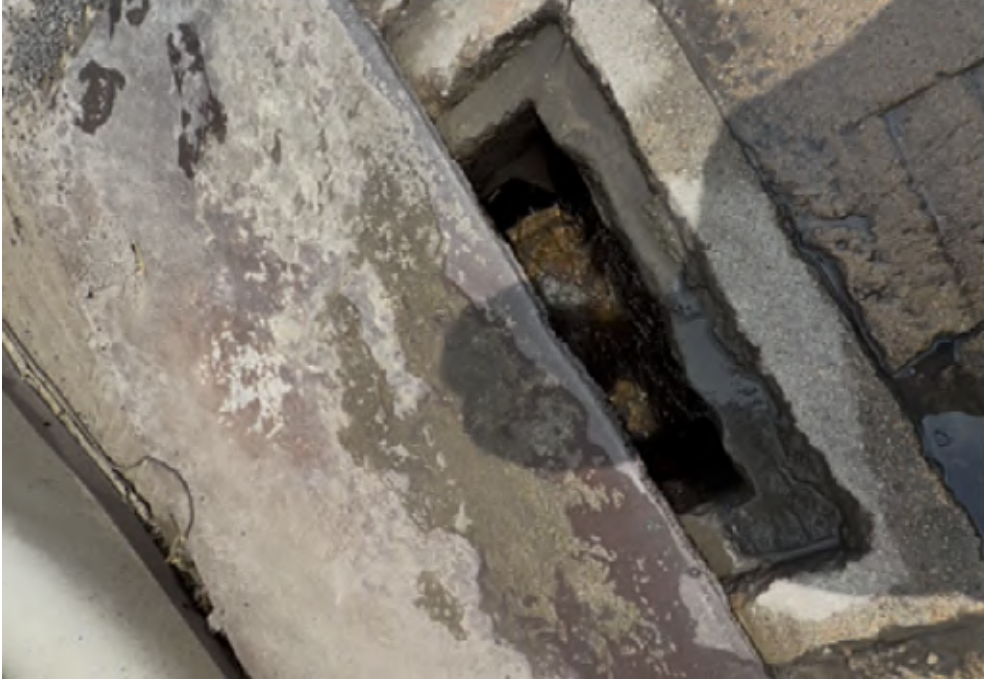
Photo e (upstream of photo 4)
