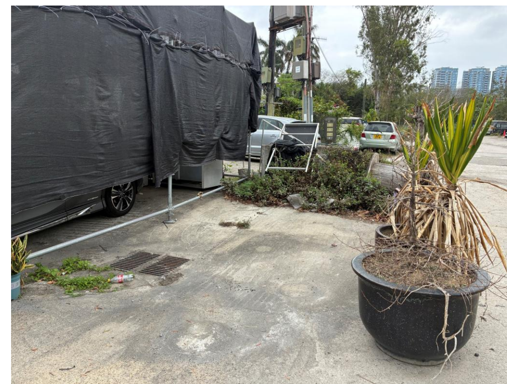
Photo 3: Drainage culvert leading to the channel
