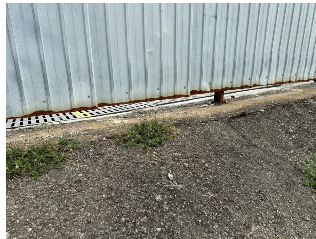
Photo 3: Perimeter U-channel at the carpark North of the site
