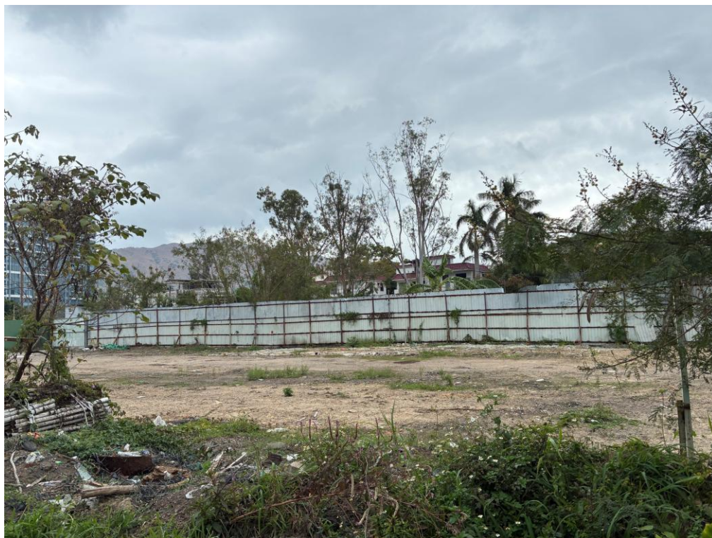
Photo 2: Fence at west of Project Site has no concrete footing
