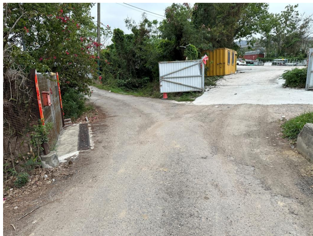
Photo 2: Trench drain at the south of the Project Site
