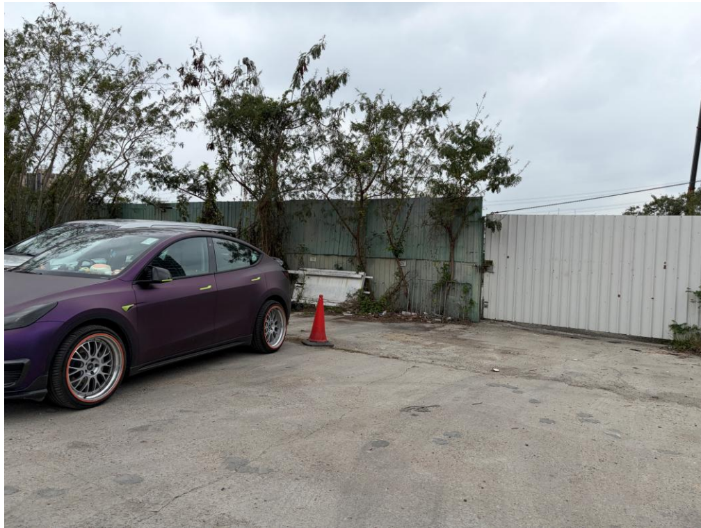
Photo 1: Fence at west of Project Site has no concrete footing
