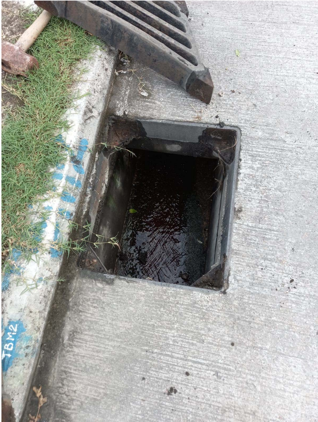
Photo 1 showing the interior of existing catchpit
