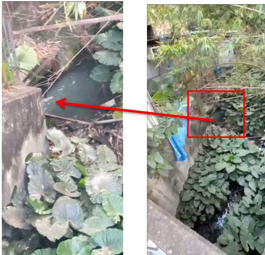
Photo 4 (Existing Village Box Culvert discharged to DSD Box Culvert)
