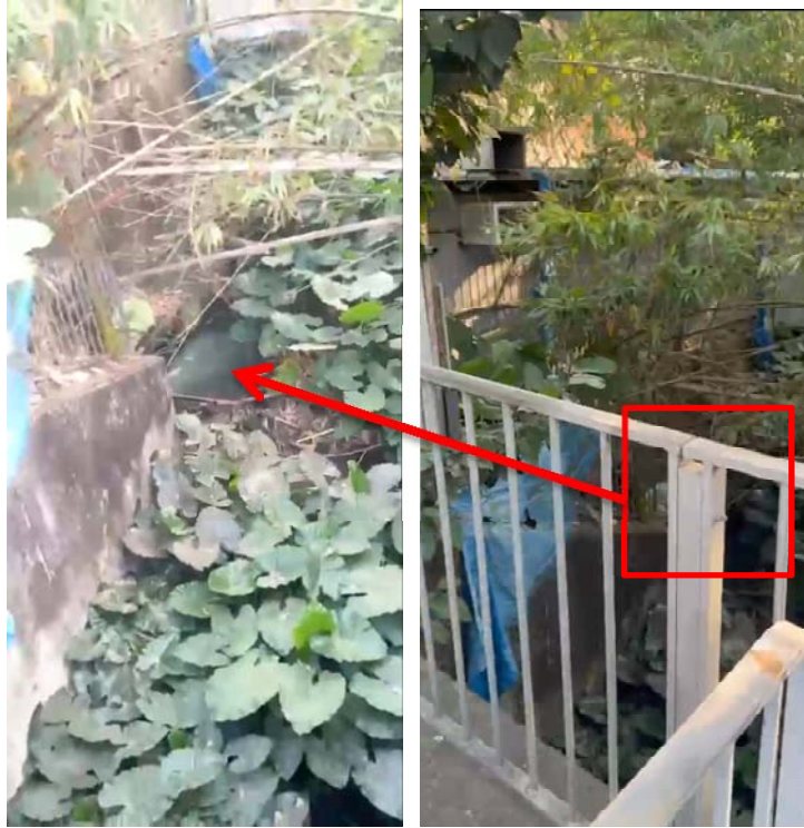
Photo 7 (Existing DSD Box Culvert)
