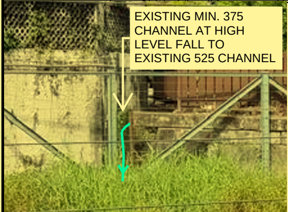
PHOTO A - EXISTING CHANNEL FALL FROM HIGH LEVEL TO LOW LEVEL
