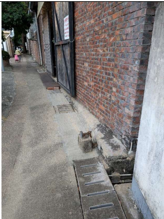
Plate 7 – Existing 225mm channel running along the eastern boundary of the Application Site flowing to the north.
