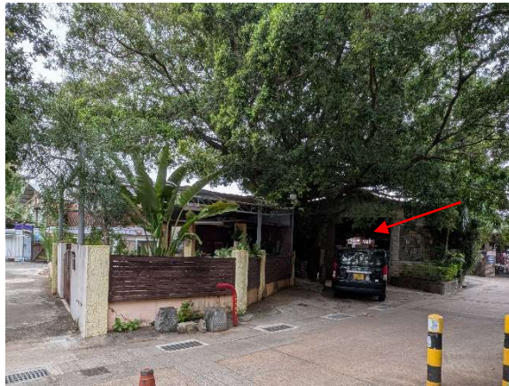
Plate 1 – Main entrance of the ‘Red Brick House’ (existing channels in front diverting surface runoff away from the Application Site).
