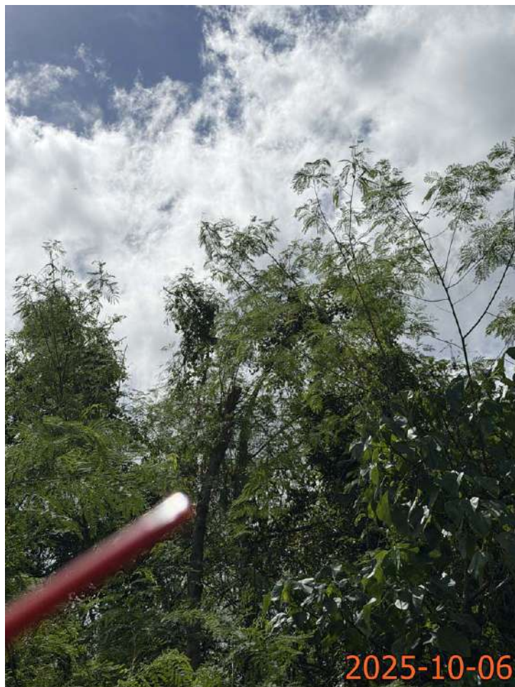
T7 Broken trunk
