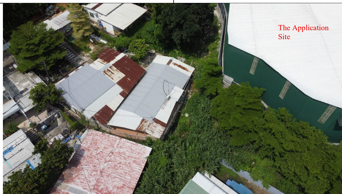
Photo No. 5 – View along the eastern boundary of the Application Site
