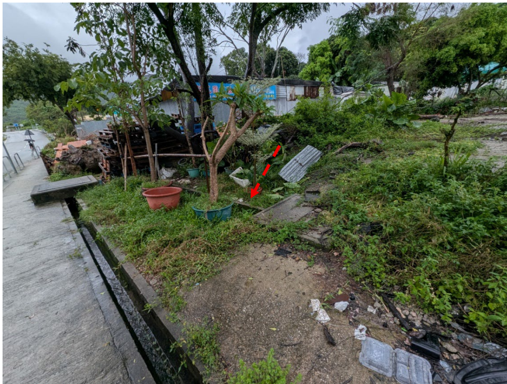
Photo No. 19 – Existing catchpit receiving flow from the existing 525 UC at Kam Ho Road
