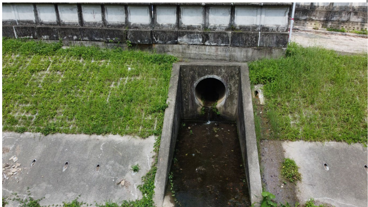
Photo No. 21 – The existing outfall at the existing 22m wide trapezoidal channel
