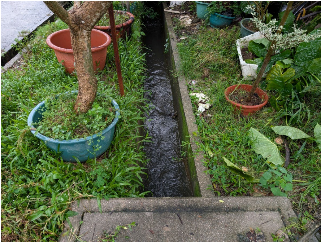
Photo No. 18 – Existing 525 UC in front of Kam Ho Road receiving the flow from the existing watercourse
