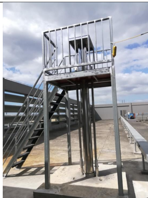
Structure for raising the Dome with Solar Tracker up to 2m high above R/F
