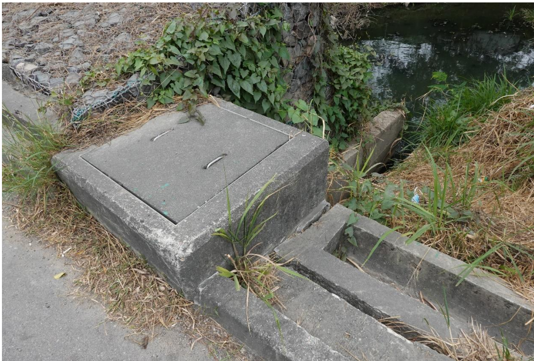
Figure 2. Existing outlet of application site
