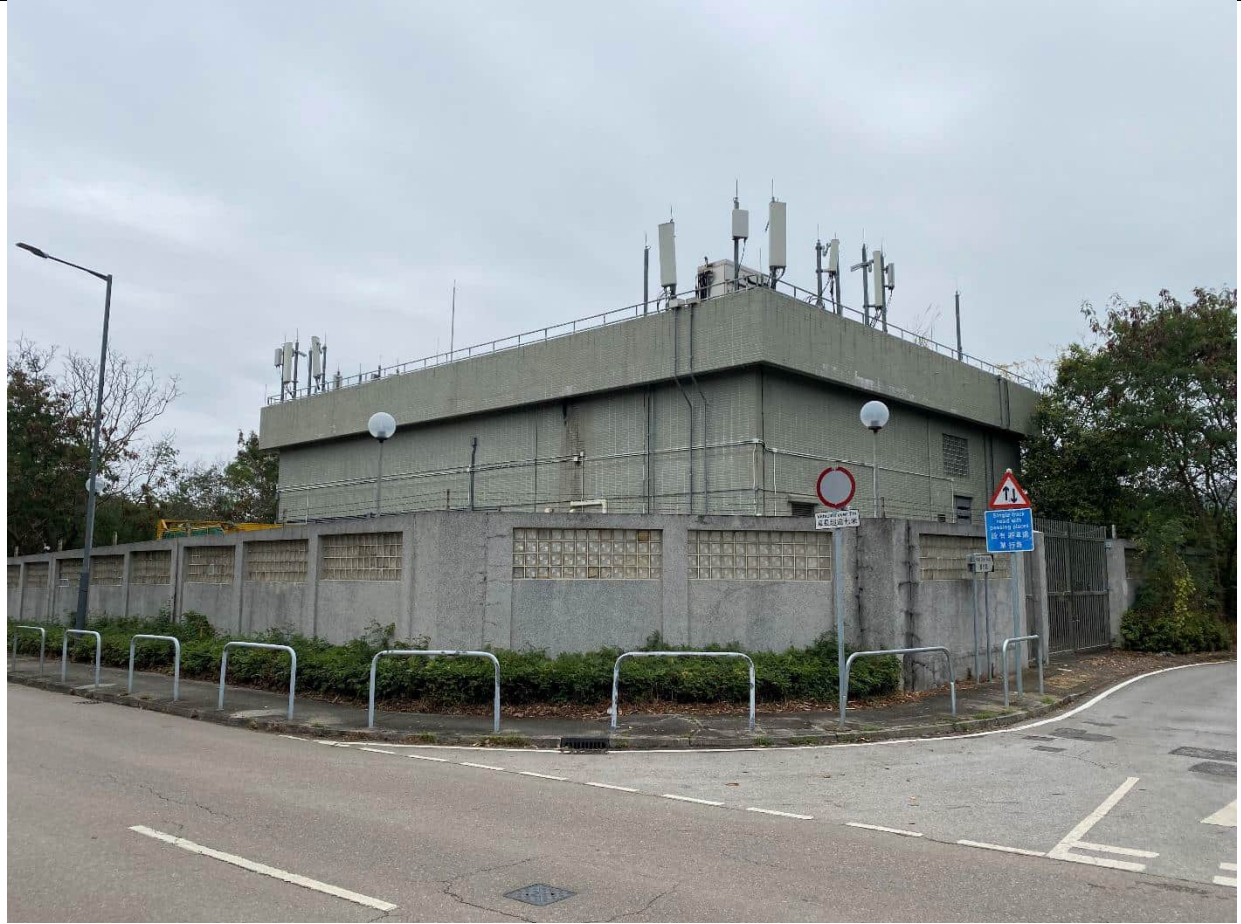
NS01: Chuk Yuen Stormwater Pumping Station
