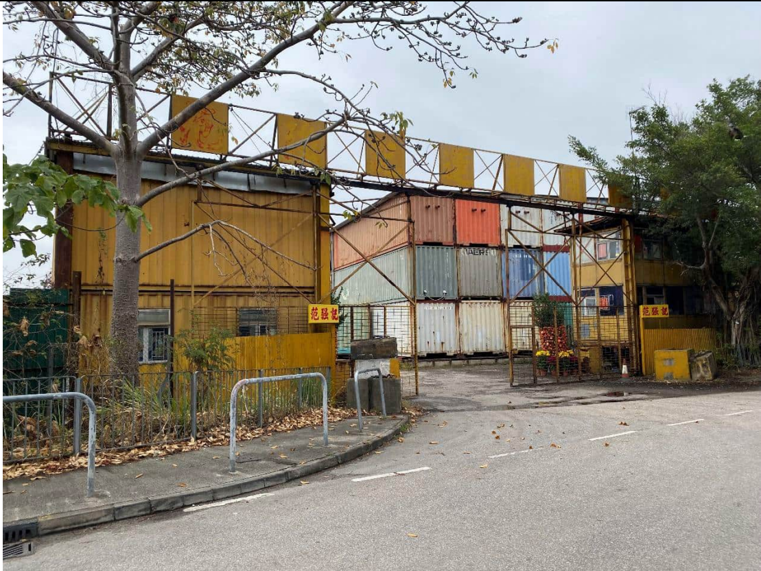
NS02: Open Storage Site with associated Warehouse (Fan Keung Kee)
