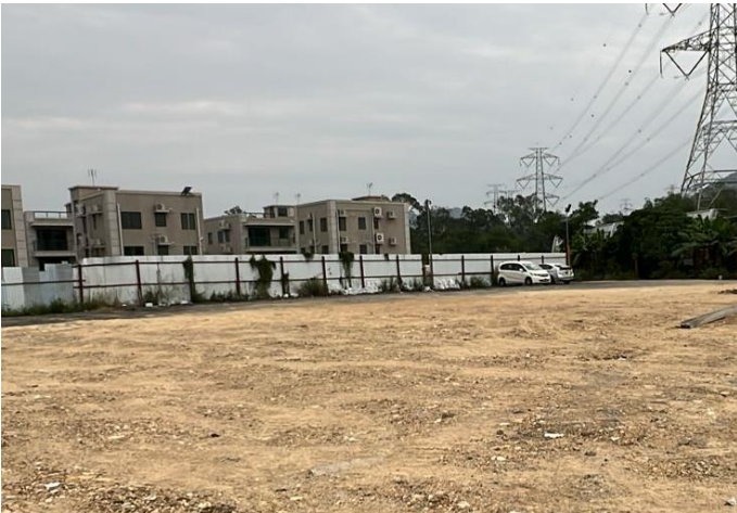
Photo 3: Site perimeter at southwest of the site
